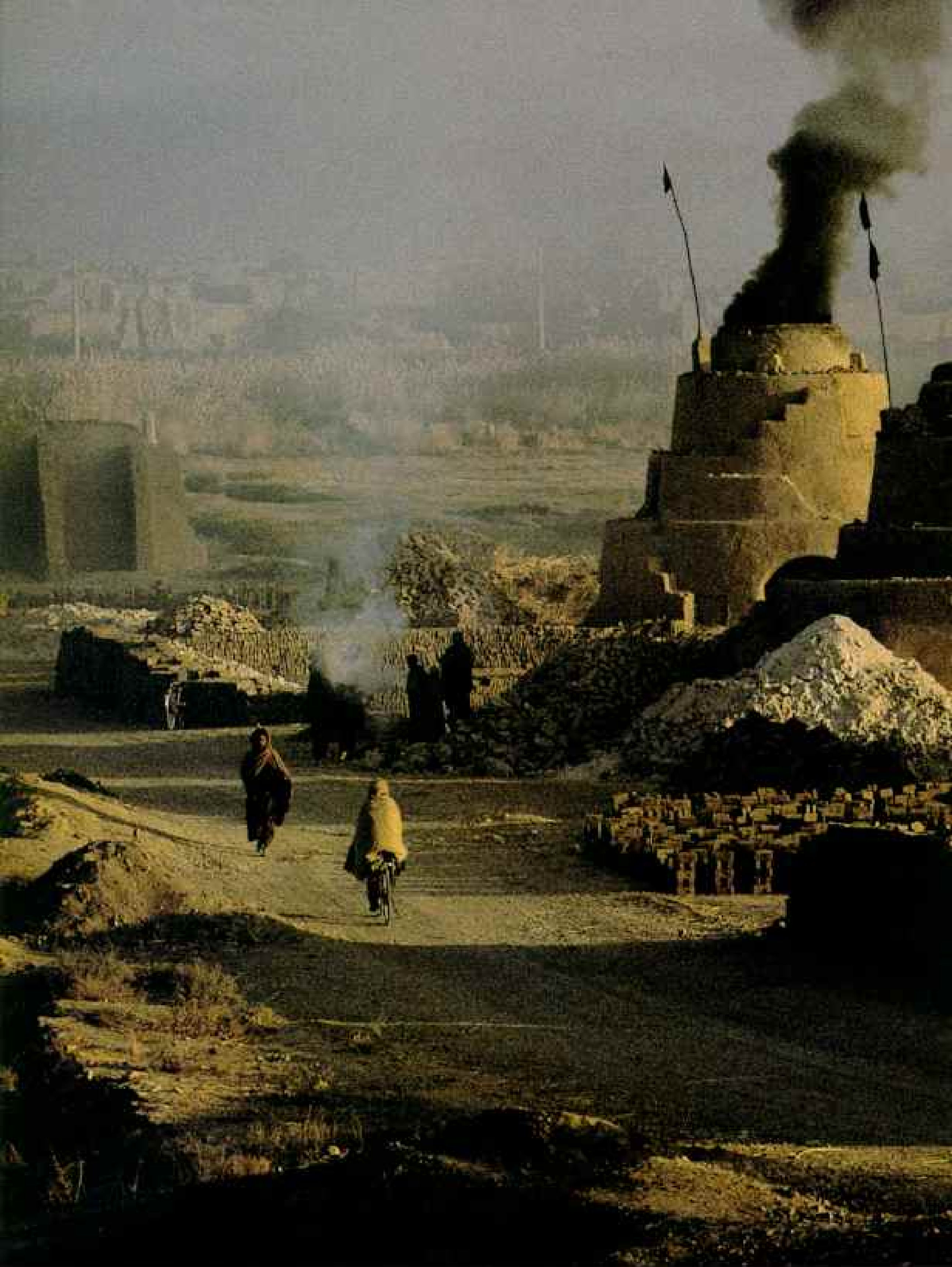
BRICK BY BRICK , residents of the southern city of Qandahar—until recently Afghanistan's largest city after Kabul—are rebuilding homes leveled by war, using bricks of soft mud fired in conical kilns outside town. Such kilns are
