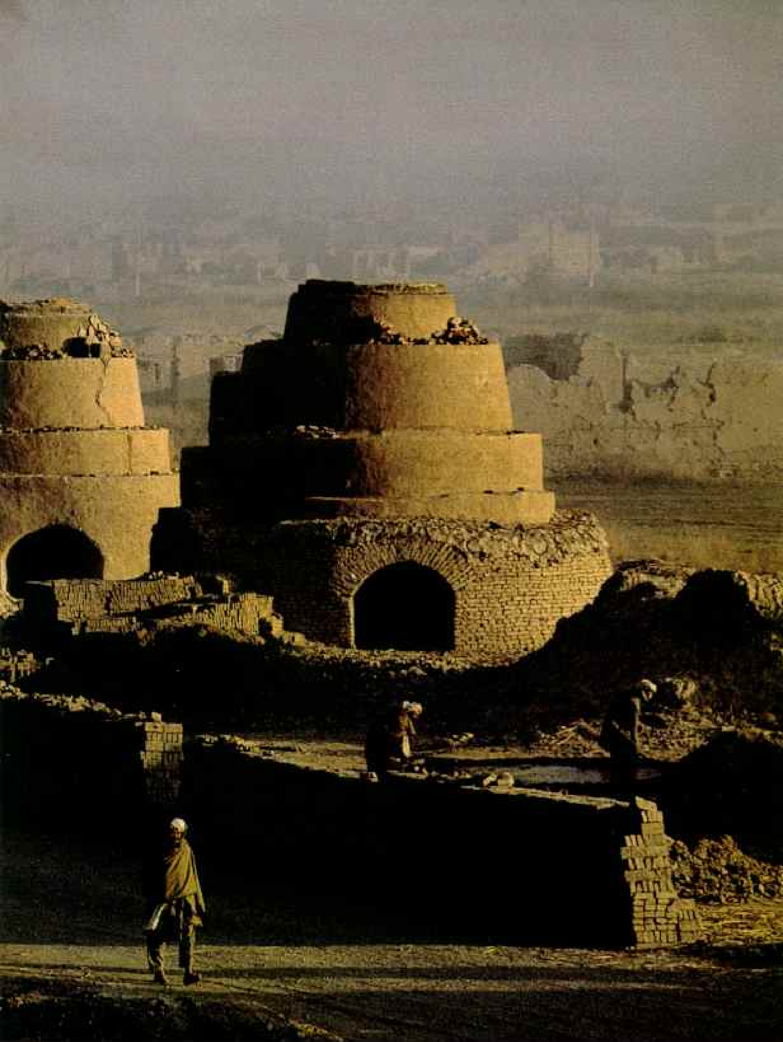
working overtime in most major cities: Two million refugees have returned to Afghanistan from Iran, Pakistan, and other points abroad, and their reconstruction efforts depend on a steady supply of bricks.
