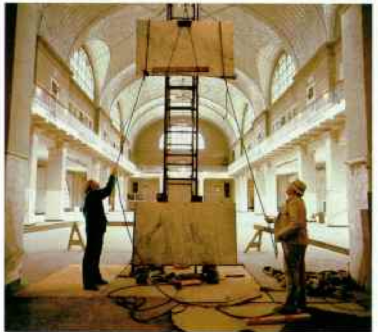
WORKERS HOIST MARBLE PARTITIONS FOR REINSTALLATION.
