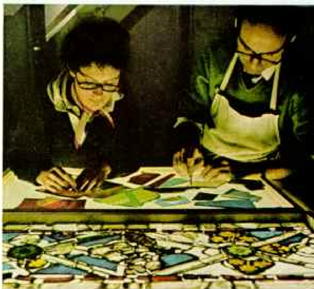
Mending time's rents, masons seal cracks in the ceiling of the Dean's Chapel (above). Restorers painstakingly cut clear glass (below) to reinforce panes in a 12th-century window. To finance the costly repairs, cathedral officials have appealed for donations of 3.5 million pounds—more than seven million dollars.
