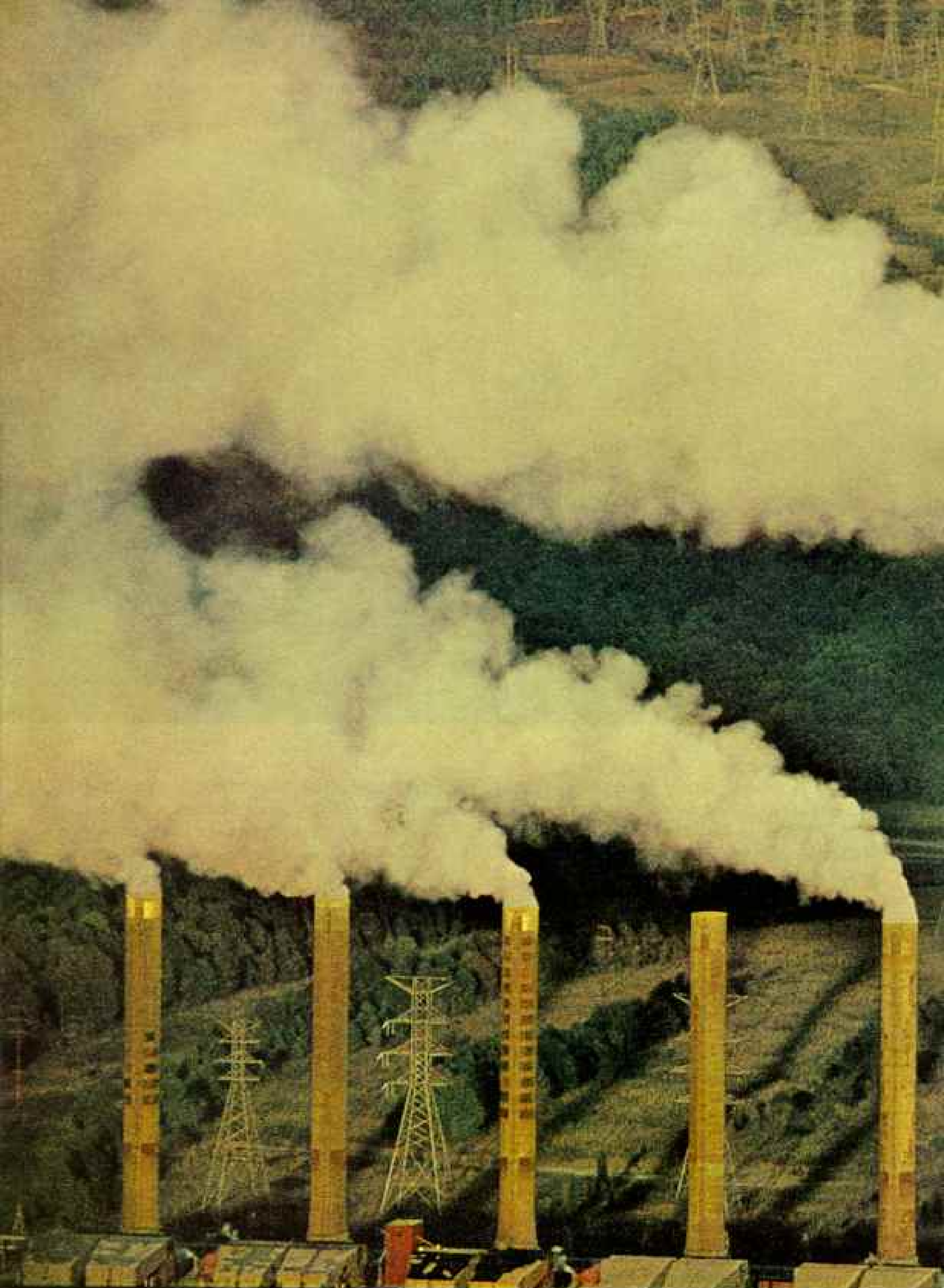
Fly ash by the ton spews from a 20-year-old coal-fueled power plant at New Johnsonville, adding to air pollution that afflicts much of the U. S. Highlines leap the hills to power-hungry
