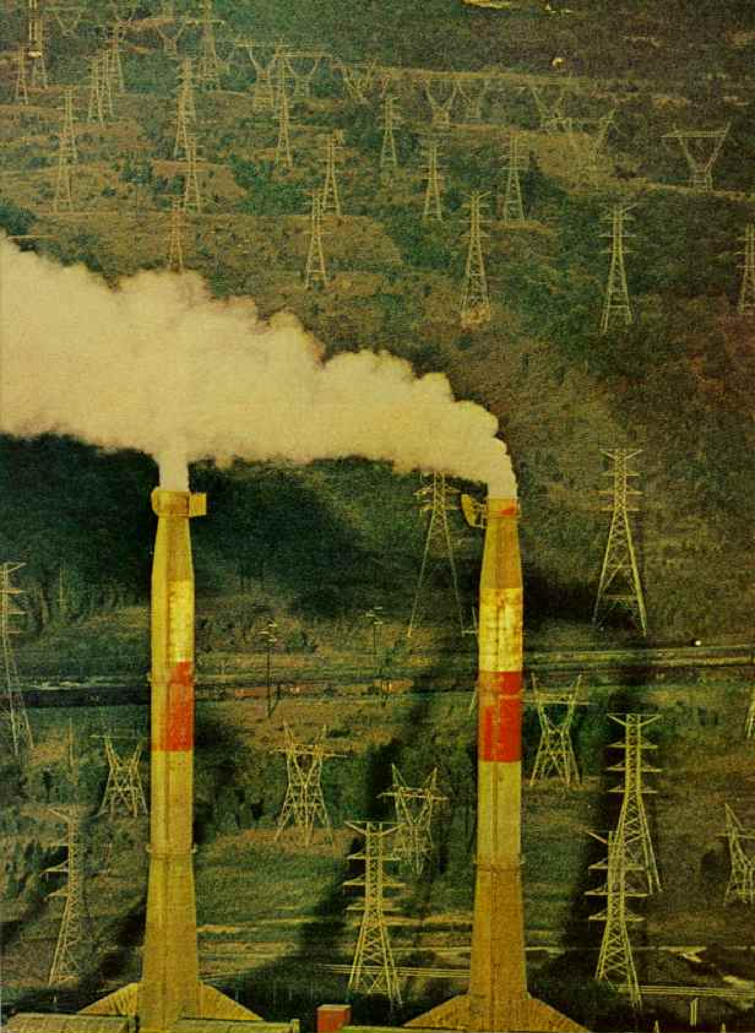
Memphis and Nashville. To cut the smoke, TVA is gradually installing electrostatic precipitators in all its coal-burning plants, but the problem of sulphur emissions remains to be solved.
