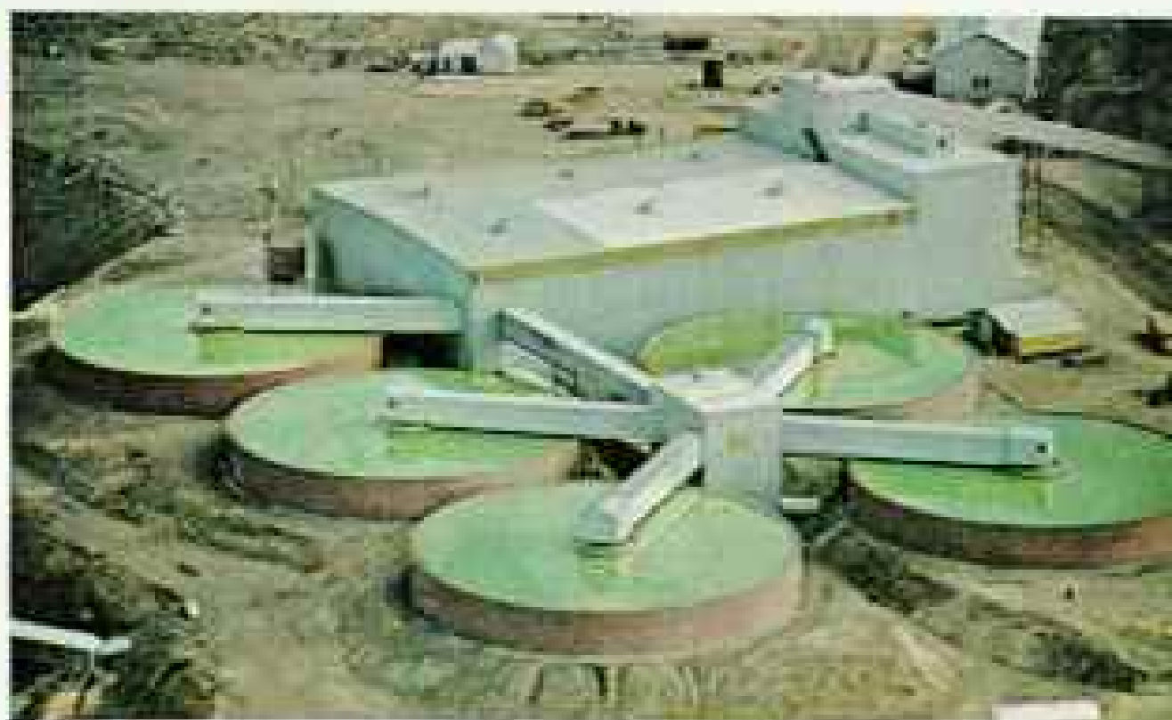
Thickener tanks settle out waste while gold-bearing cyanide, called pregnant solution, flows off the top.
