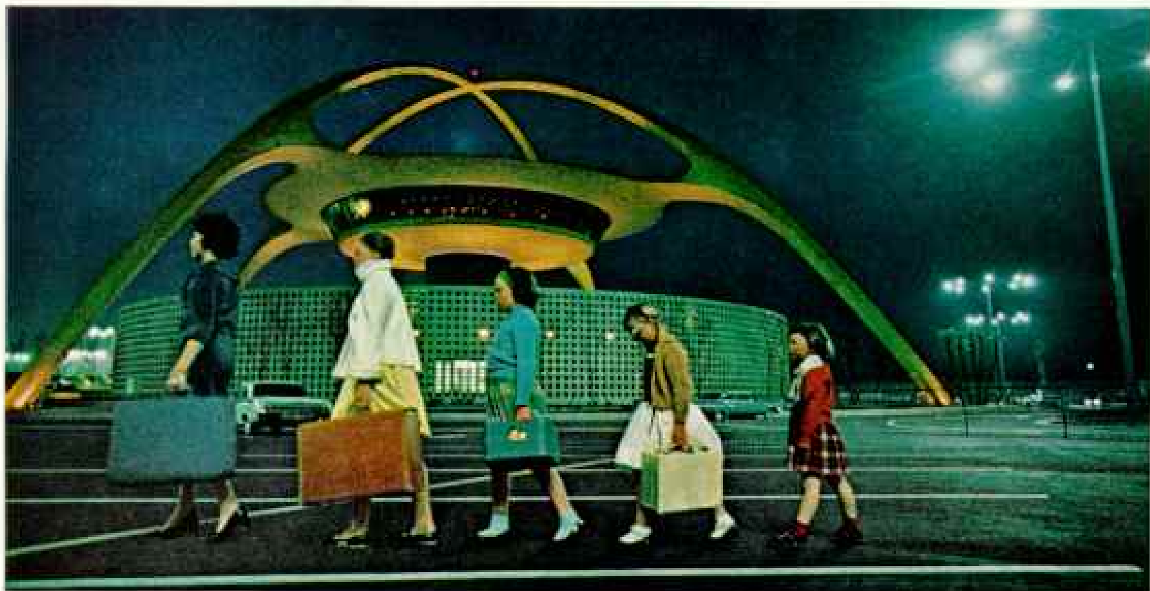
Graceful parabolic arches dome a restaurant in the sky at new Los Angeles International Airport.
