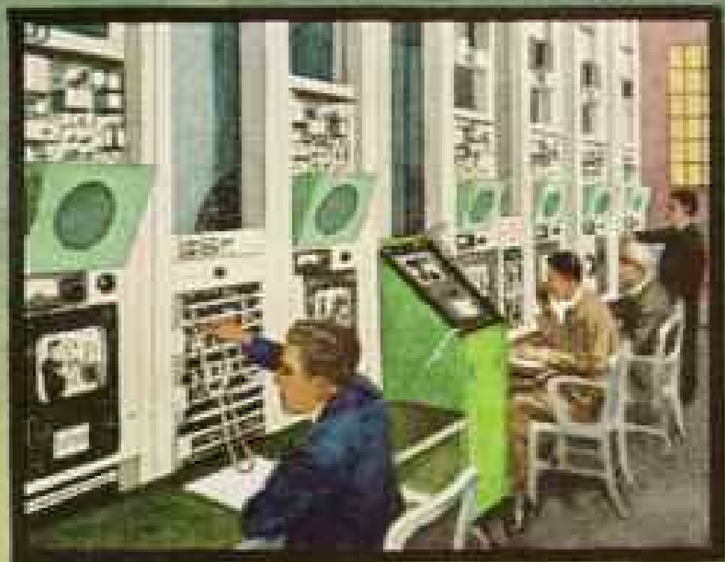
3. A. T. & T. Network Control Room. Telephone channels are set up here to carry TV signals across the country.
