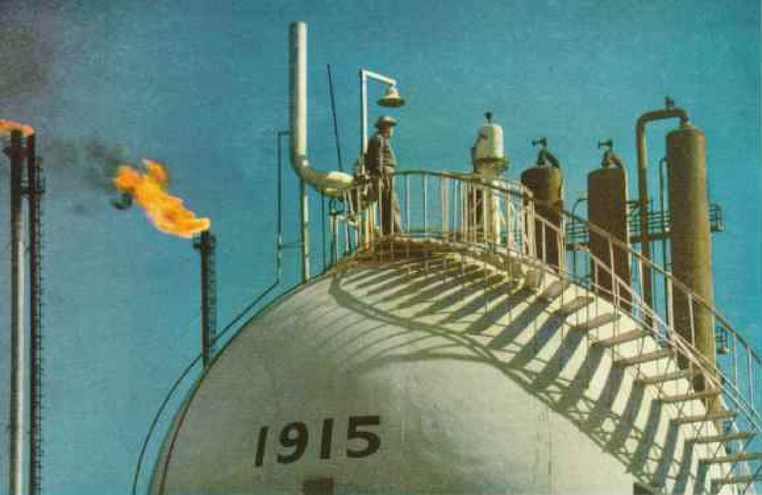
This Standard Oil Sphere at Baton Rouge Holds Isobutylene for Synthetic Rubber
