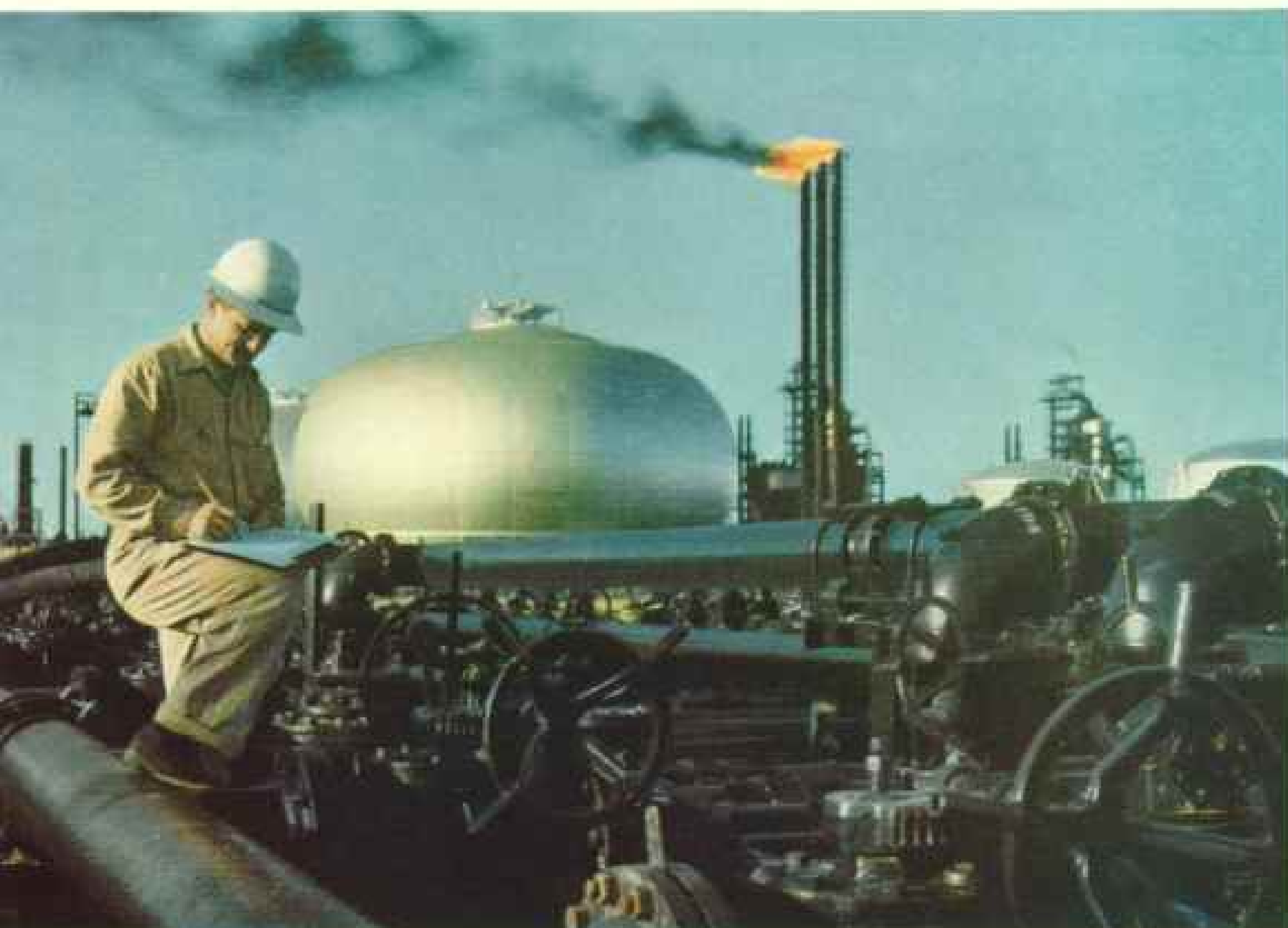
This Standard Oil Sphere at Baton Rouge Holds Isobutylene for Synthetic Rubber
