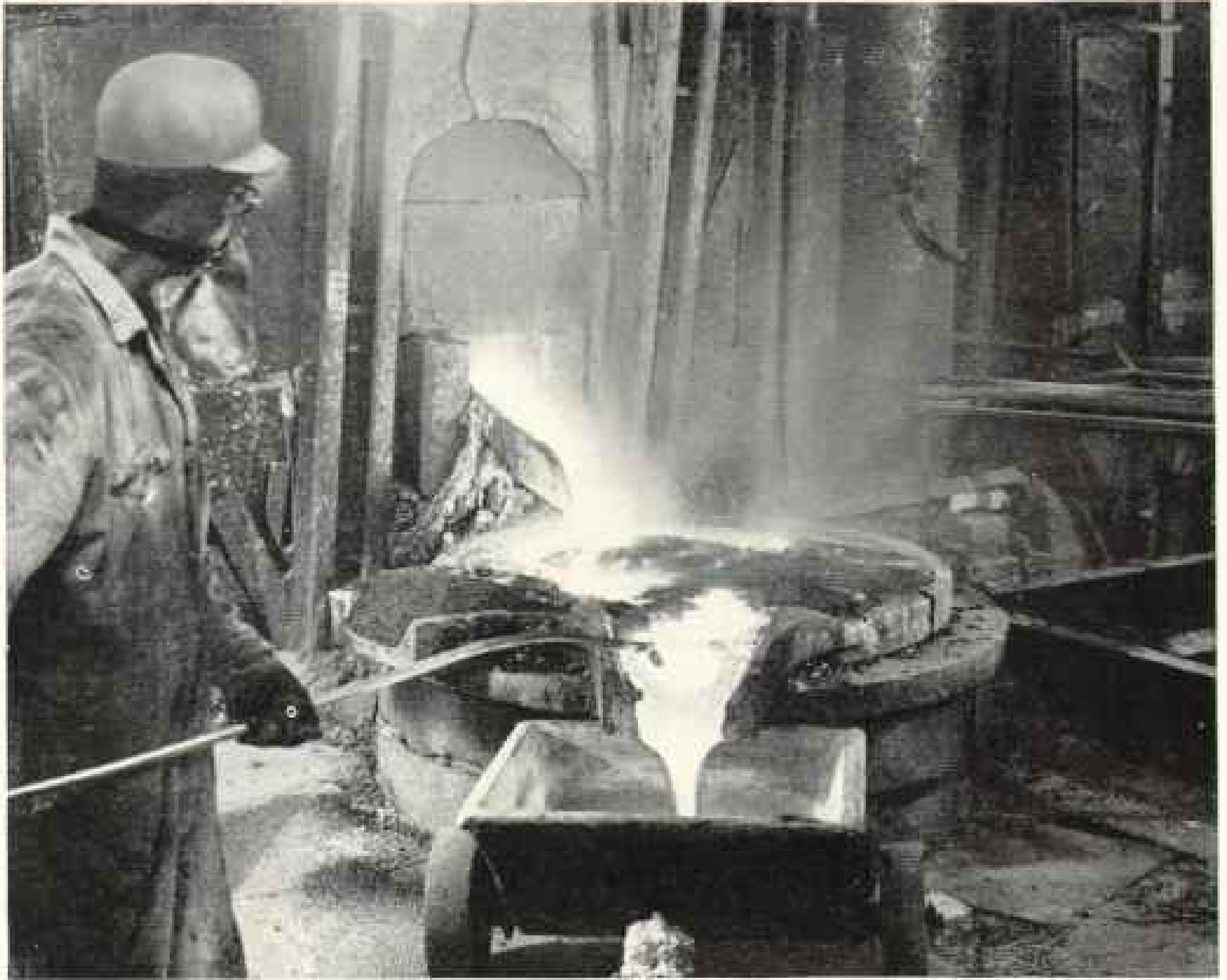
MELTING SCRAP LEAD from discarded telephone cable. It is melted and refined at a Western Electric plant. The lead ingots will return to service as new cable sheathing.
