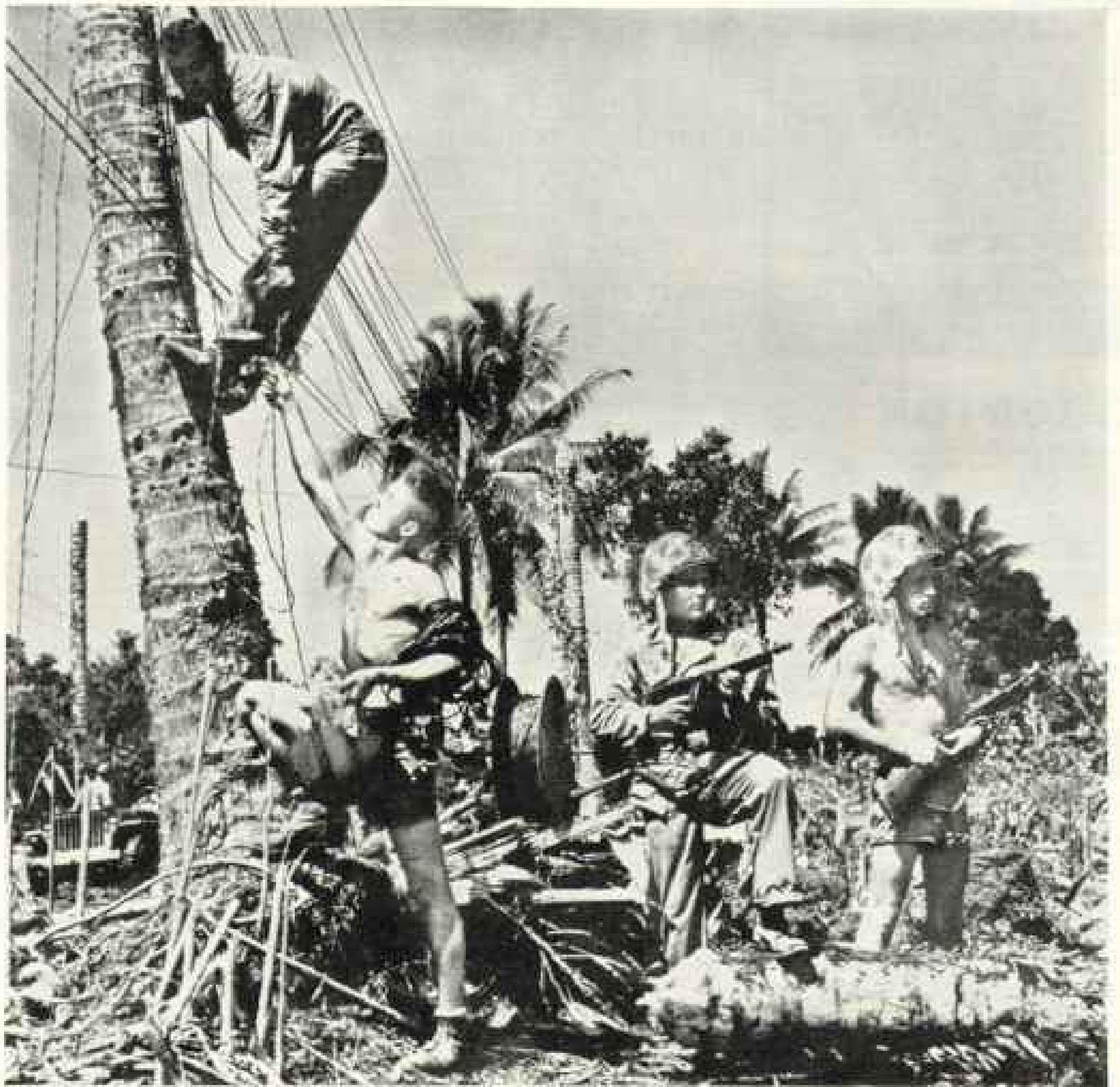
U. S. MARINES ON BOUGAINVILLE use palm trees for telephone poles as they string communication lines. Two stand guard.
