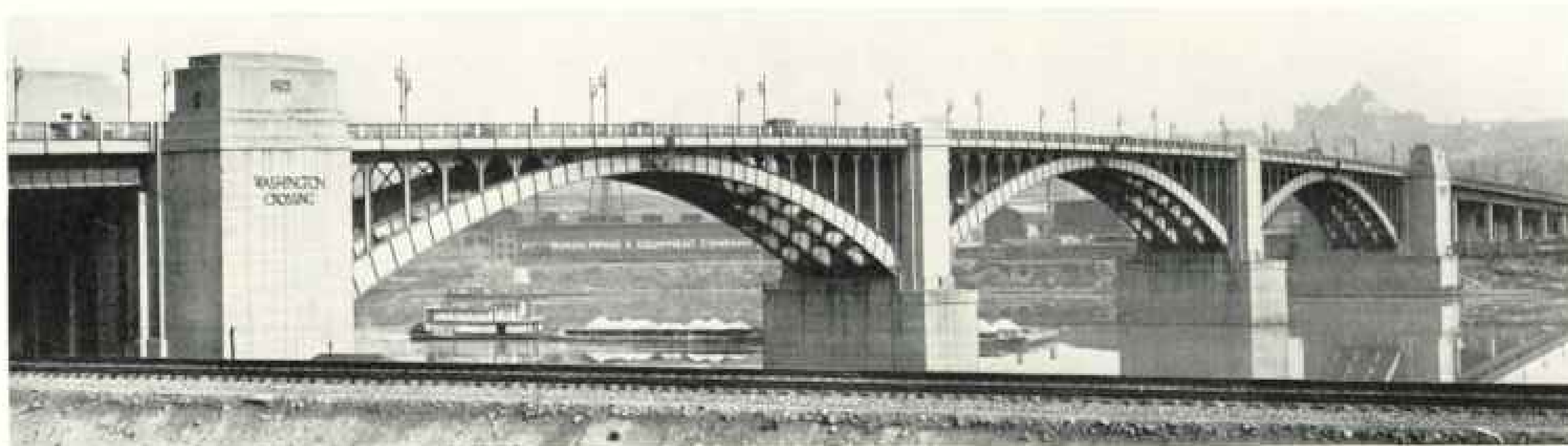
THE WASHINGTON CROSSING BRIDGE SPANS THE ALLEGHENY RIVER WHERE MAJOR WASHINGTON NEARLY LOST HIS LIFE RETURNING FROM FORT LE BOEUF (SEE TEXT, PAGE 18)
