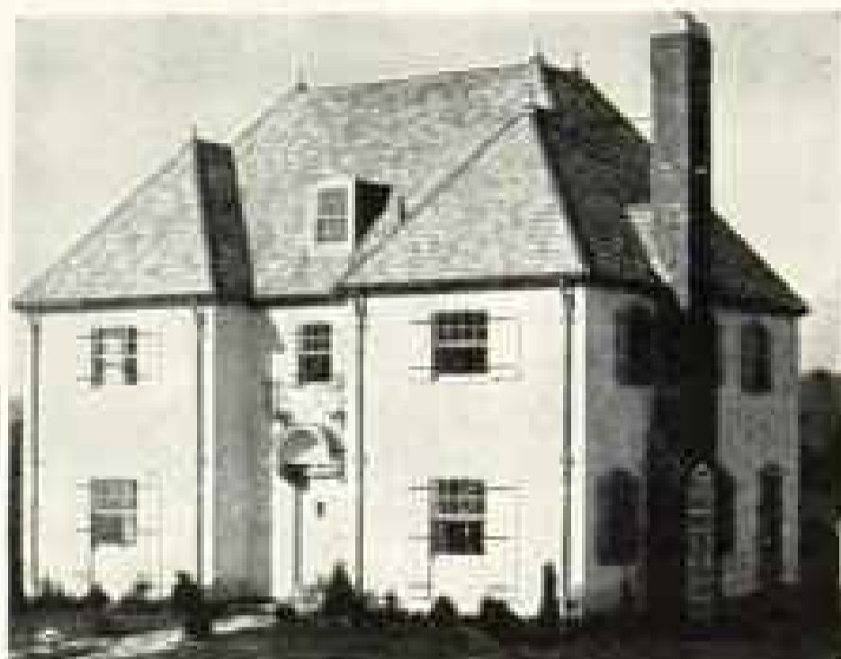
Johns-Manville Colothlene Asbestos Shingles on a residence at Worcester, Mass. Designed by Harold J. Beaudette. Shingles furnished by W. H. Sawyer Lumber Co.
