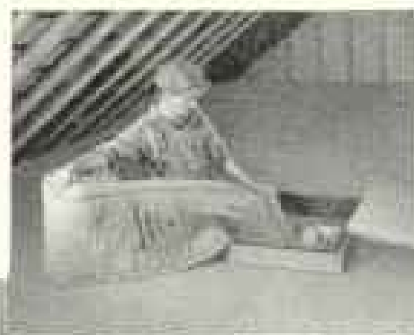
Balsam-Wool can easily be carried through any opening that will admit the body of a workman. Strips of Balsam-Wool cut to proper length in the basement or garage can be carried to the attic by a single workman.
