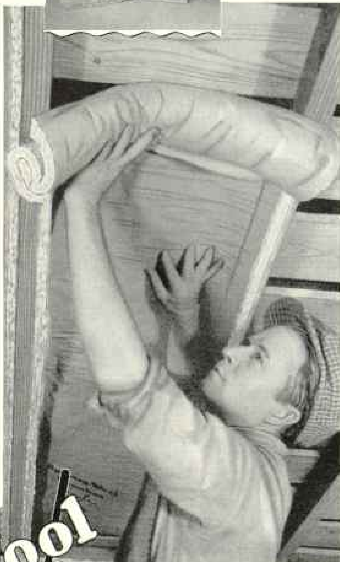
Balsam-Wool can easily be carried through any opening that will admit the body of a workman. Strips of Balsam-Wool cut to proper length in the basement or garage can be carried to the attic by a single workman.
