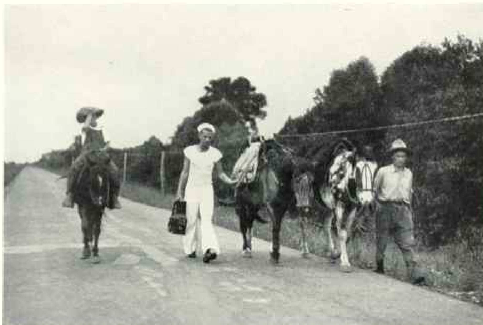
AN EXCELLENT SPECIMEN OF AMERICAN-BUILT HIGHWAY THROUGH A CANAL ZONE SWAMP
