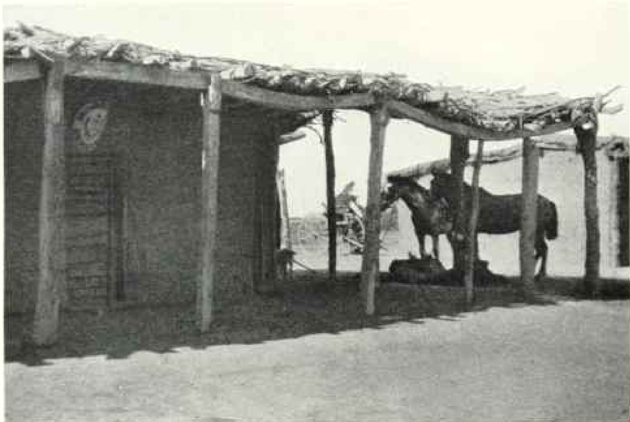
A COUNTRY POLICE STATION IN THE PROVINCE OF SANTIAGO DEL ESTERO, ARGENTINA. The buildings are constructed of quebracho poles, covered with reeds and mud. The author's horses are tied under the shed.
