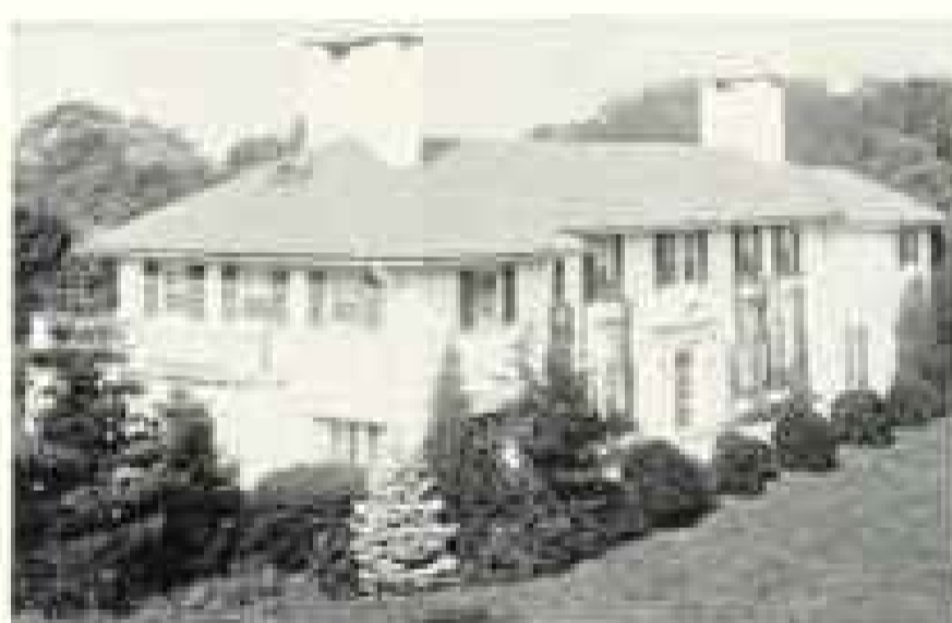
Attractive home of Geo. E. Smith, at Great Neck Estates, Long Island, N. Y. Its architect—W. Albert Swasey. Roofed with J-M Asbestos Shingles.
