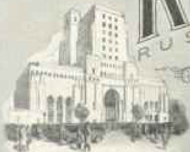
R. P. O. B. Building, Los Angeles, Calif. Architect—Carter & Johnson Contractor—Harrison Construction Co. Russwin Dealer—Russwin Hardware & Supply Co., Inc.
