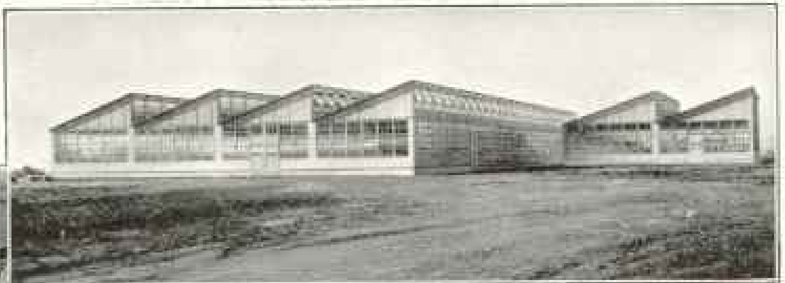
Exterior View Truscon Standard Building, Saw-tooth type McGill Manufacturing Company, Valparaiso, Indiana.
