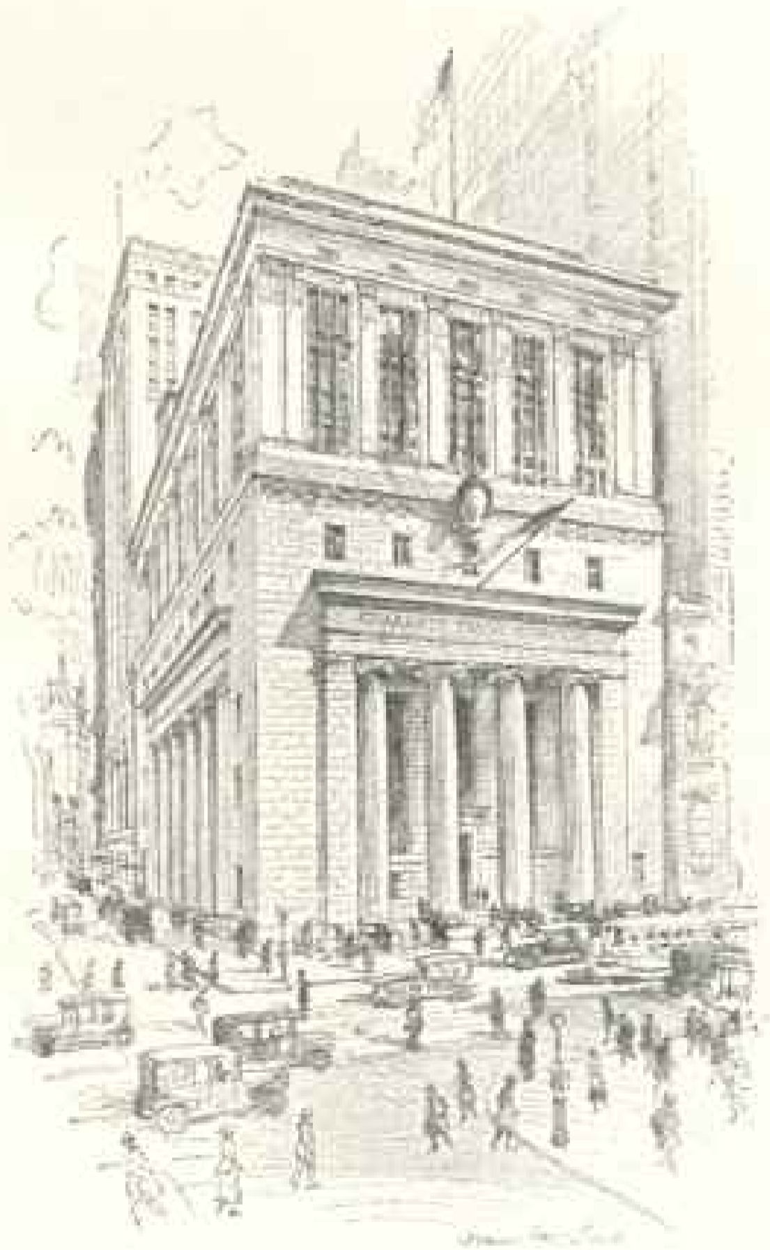
MAIN OFFICE OF THE COMPANY 140 BROADWAY, NEW YORK CITY
