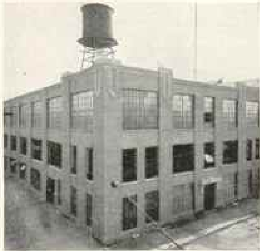
We built this building, Austin Standard No. 9 mill-type construction, 80 ft. x 408 ft., 3 stories, for the Pittsburgh Transformer Co., Pittsburgh, in 78 working days, finishing the building proper several days ahead of schedule.
