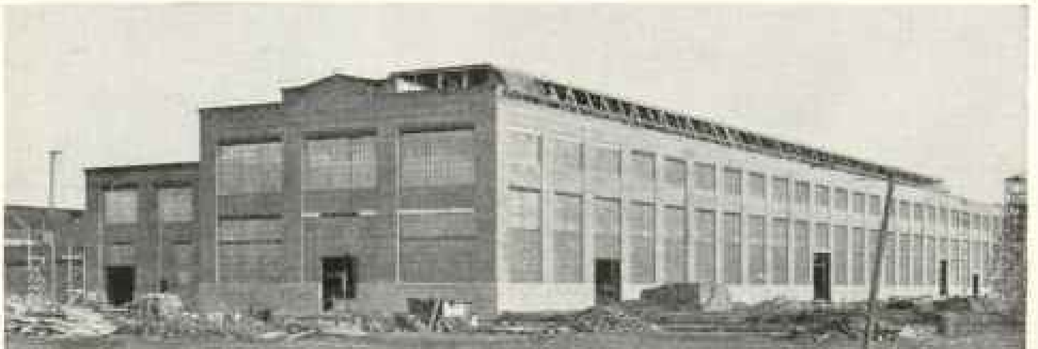
This laundry building, 120 ft. x 480 ft., for the General Electric at Schenectady, contracted for an 60-working-day schedule, was completed one week ahead of time.
