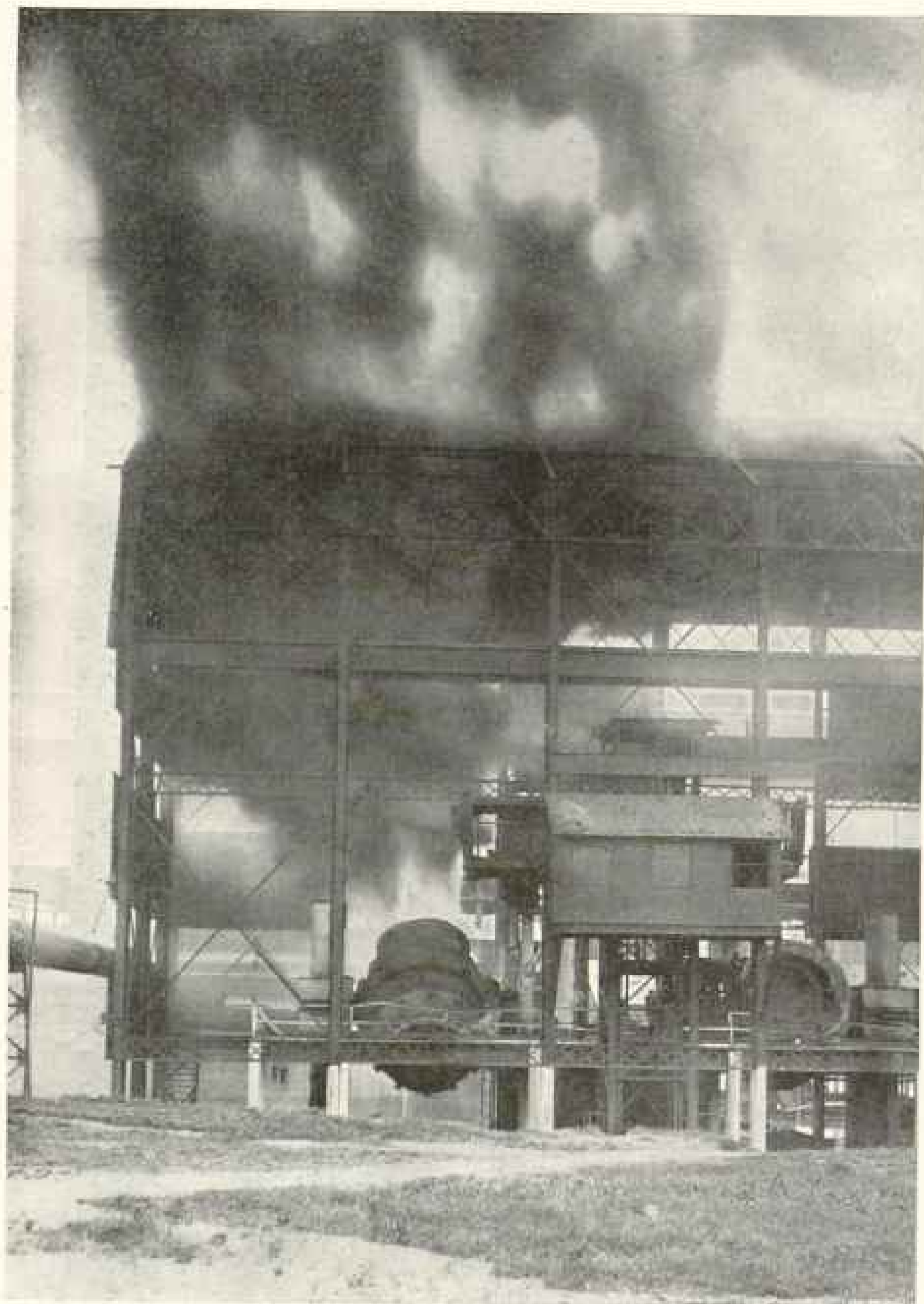
BESSEMER CONVERTERS AT WORK
