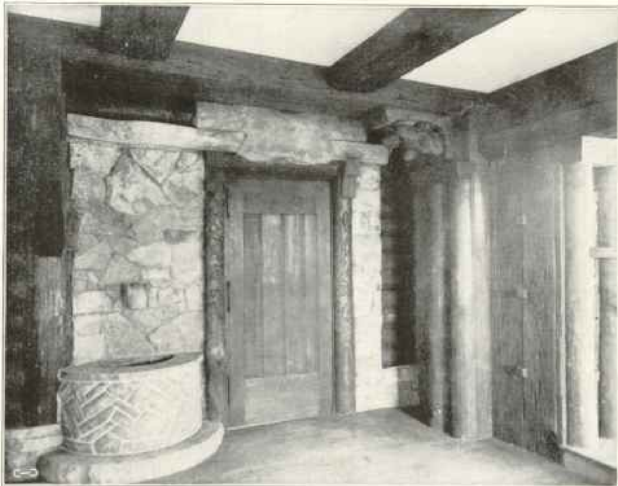
ANOTHER CORNER IN THE “FIELD” ROOM, ESTATE OF HENRY FORD, ESQ., DEARBORN, MICHIGAN. MR. W. H. VAN TINE, ARCHITECT, DETROIT.
