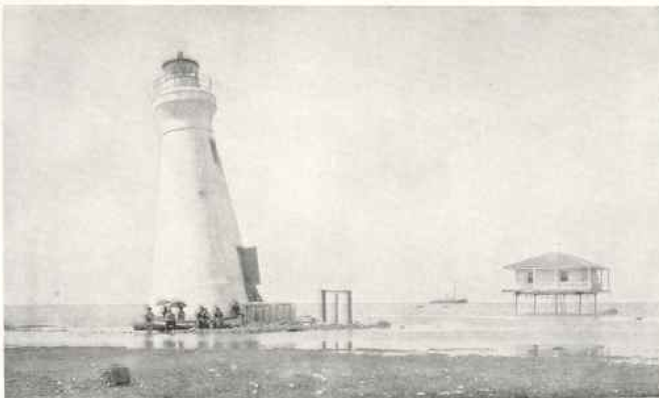
THE CHANDELEUR LIGHT-TOWER, LOUISIANA, WHICH WAS ABANDONED AFTER BEING UNDERMINED BY A TORNADO IN 1893
