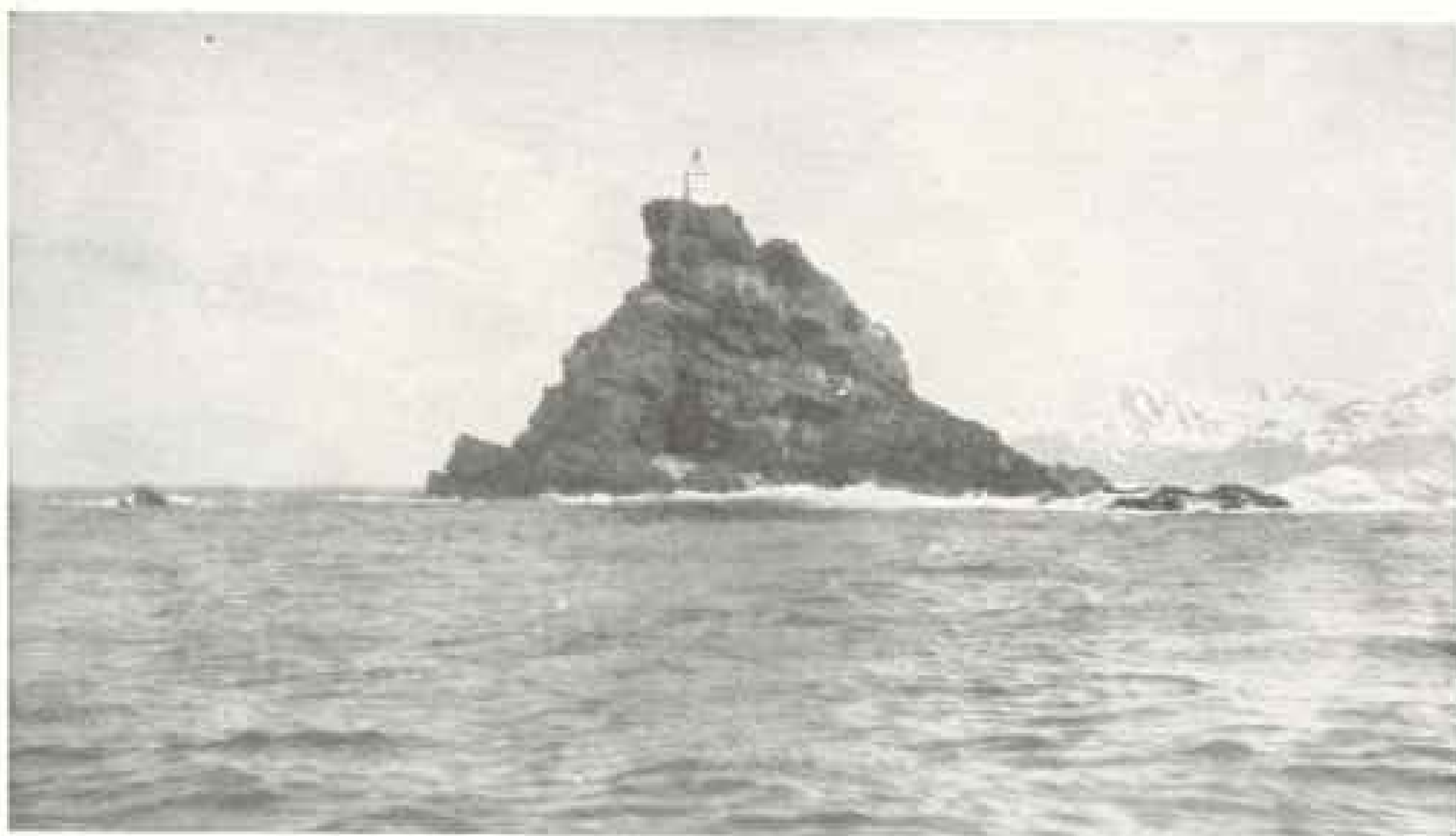
AN UNATTENDED FLASHING LIGHT AT THE ENTRANCE TO PRINCE WILLIAM SOUND! THE ZAIKOF POINT LIGHT STATION, ALASKA (SEE PAGE 35)
