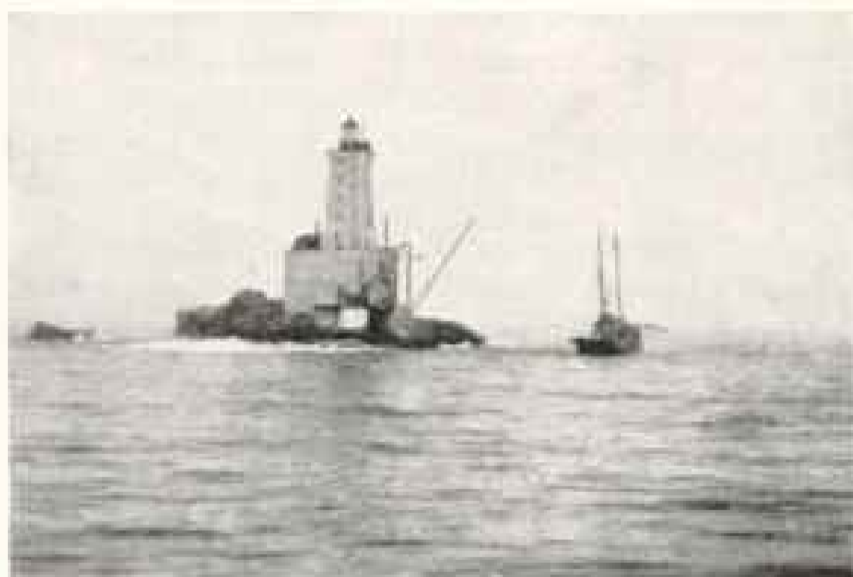
ST. GEORGE REEF LIGHT, CALIFORNIA, COMPLETED: A DIFFICULT AND EXPENSIVE STRUCTURE
