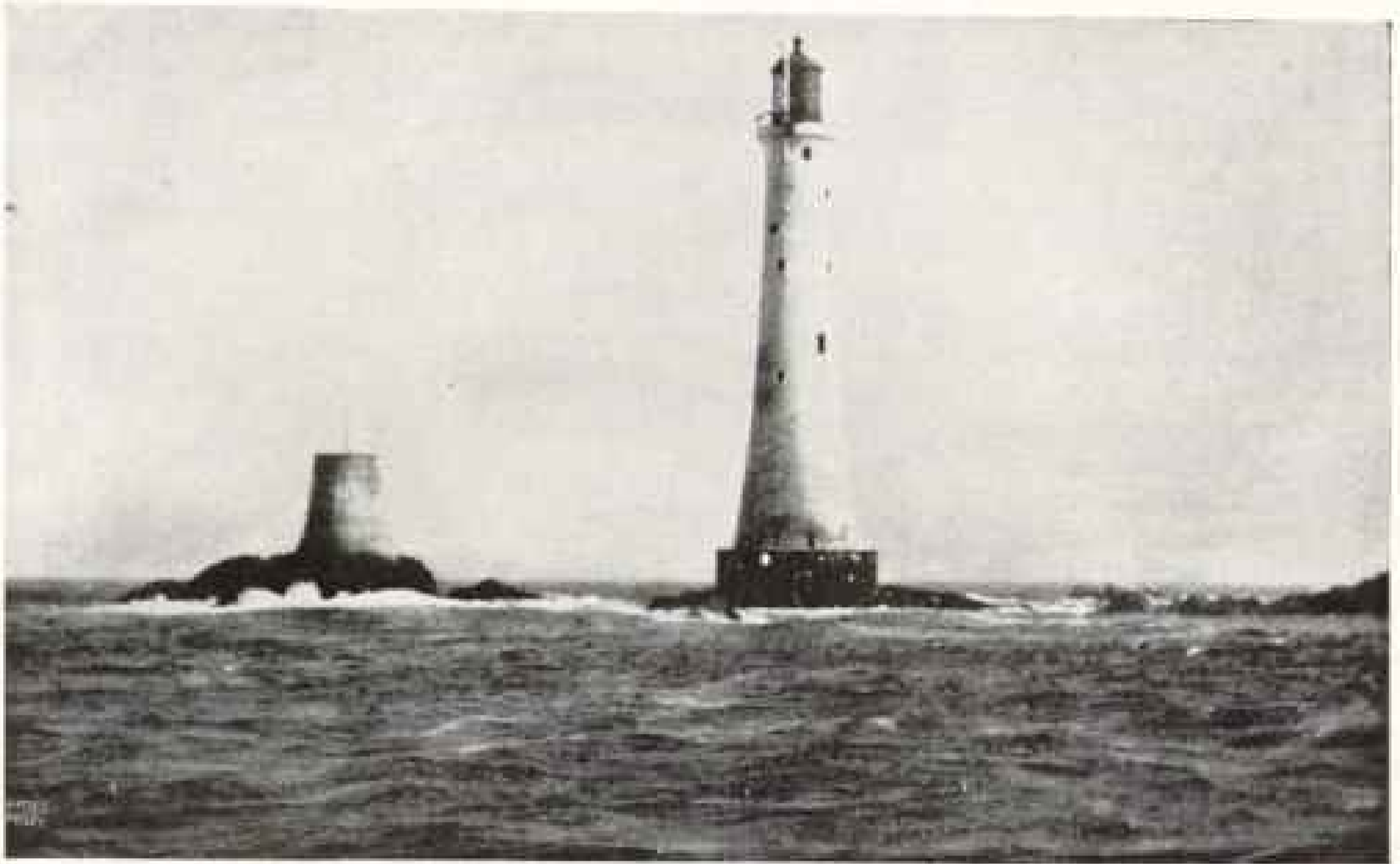
THE FOURTH AND PRESENT EDDYSTONE LIGHTHOUSE, COMPLETED IN 1881 (SEE PAGE 17)
