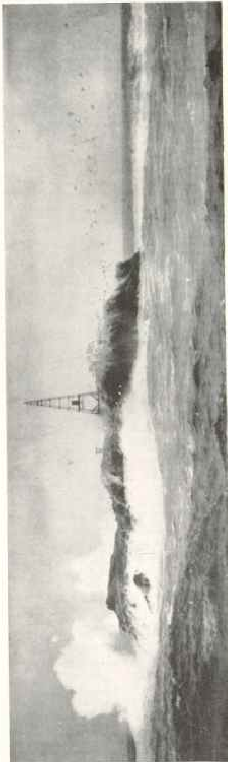
AN UNATTENDED FLASHING GAS-LIGHT ON RICHARDSON'S ROCK, CALIFORNIA
