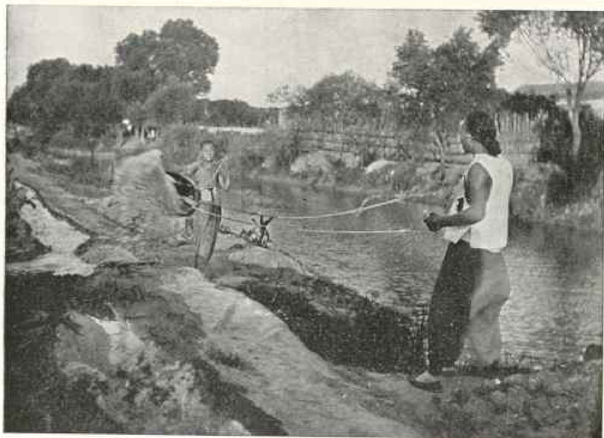
THE YOUNG MAN IS LOADING HIS BOAT WITH CANAL MUD, USING THE LONG-HANDLED CLAM SHELL DREDGE, WHICH HE CAN OPEN AND CLOSE AT WILL. IRRIGATION BY MEANS OF THE SWINGING BASKET, PROVINCE OF CHI-LI, CHINA
