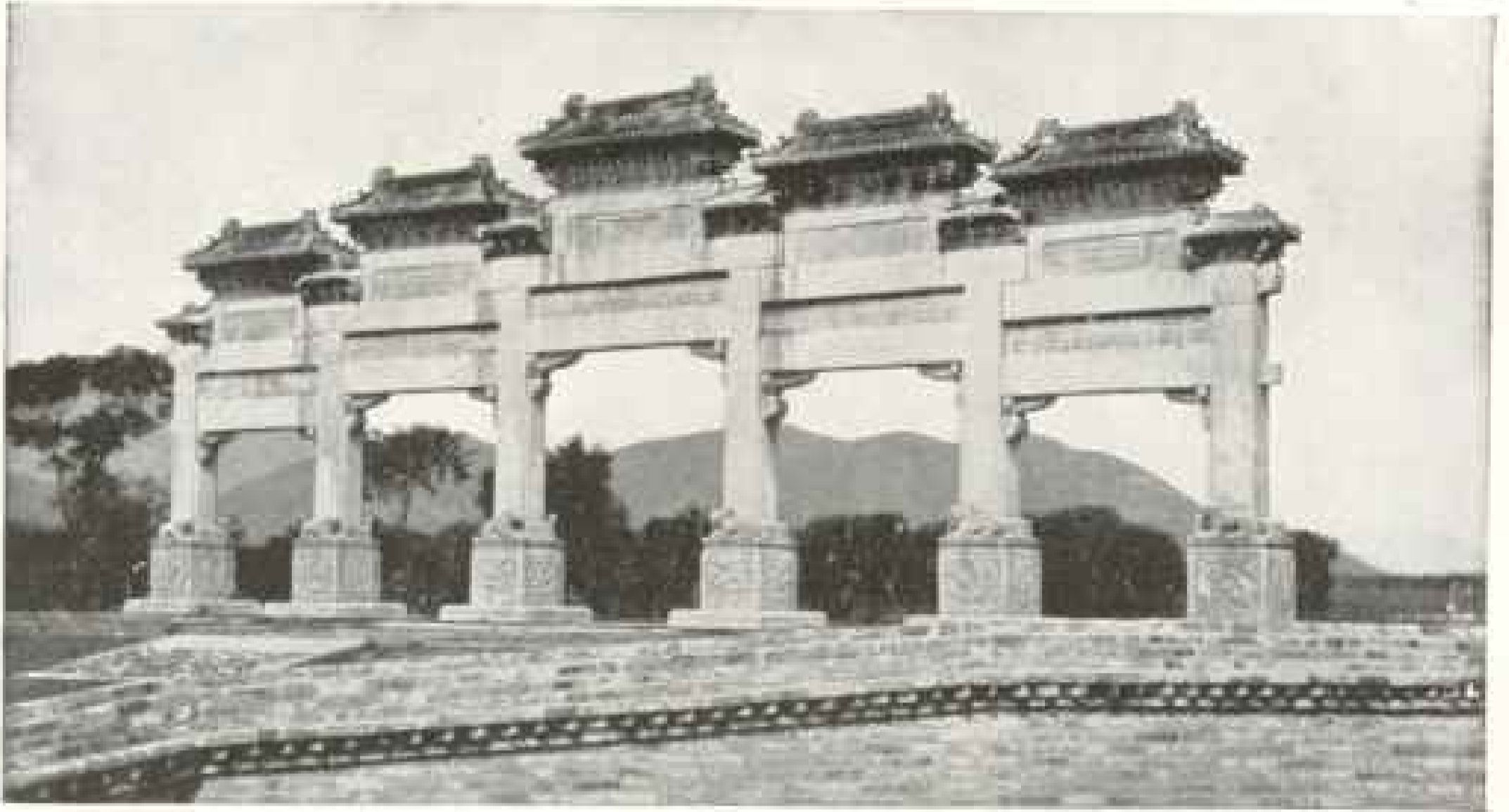
THE FIVE-ARCHED P'AI-LOU AT THE ENTRANCE TO THE "HOLY WAY," IN THE VALLEY OF THE MING TOMBS (SEE TEXT, PAGE 1000)
