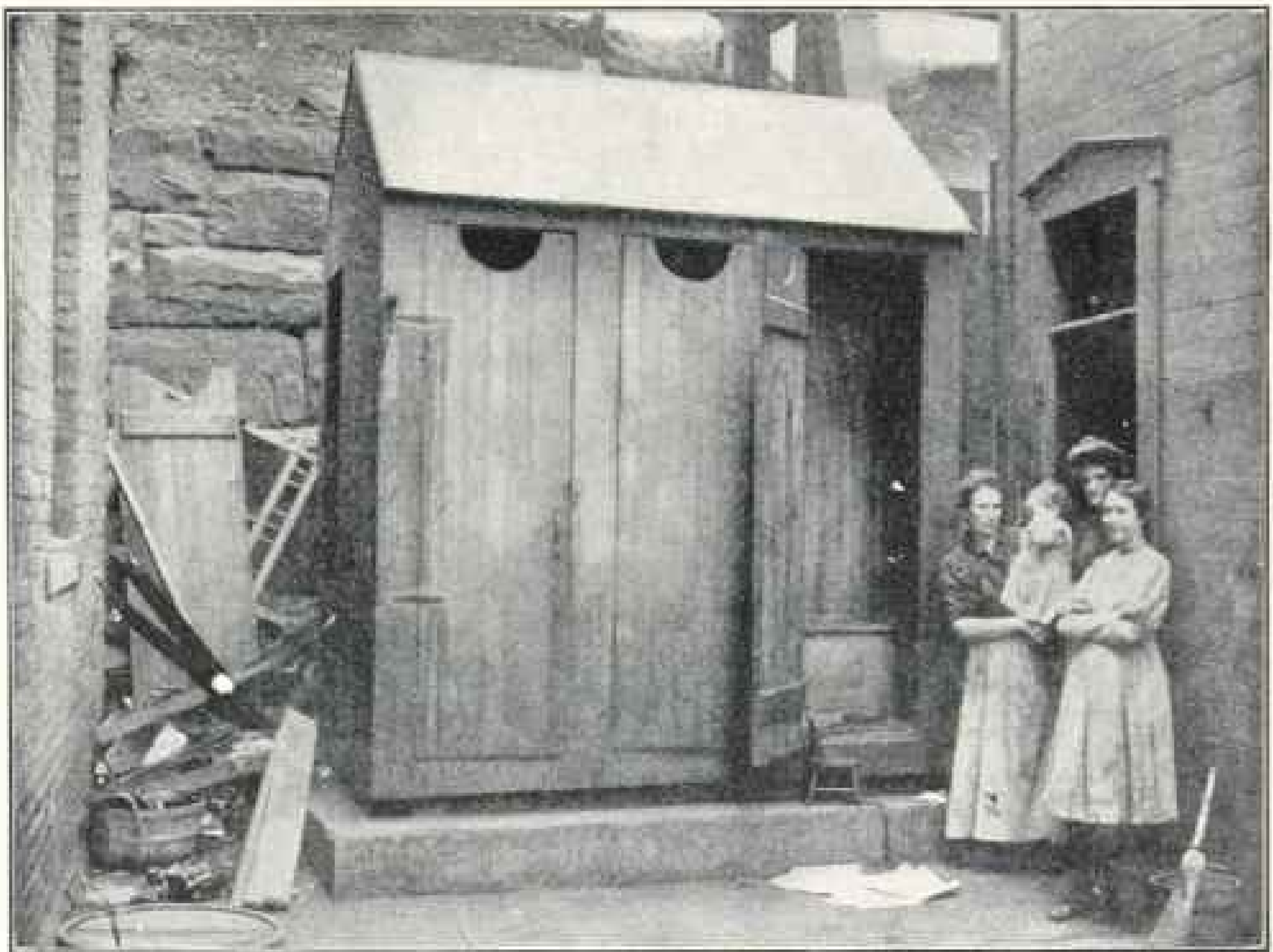
PRIVY VAULTS, SWARMING WITH FLIES, ADJOINING KITCHEN DOOR
