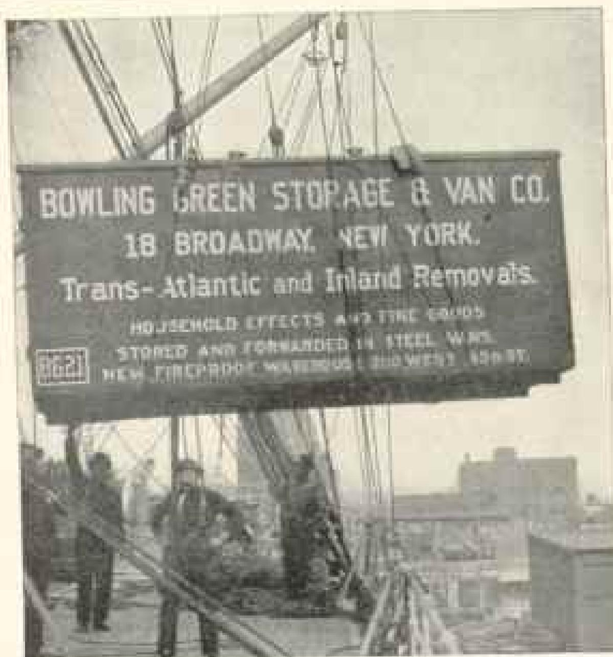
HOISTING LIFT-VAN ON BOARD STEAMSHIP
