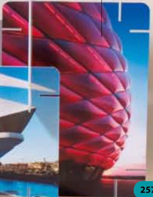
Some 3,000 air-filled foil panels that form the exterior can be lit from within to match the home team's colors
