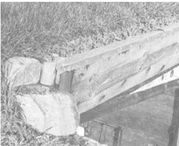
Illus. 15-2. Removing the sod within 5" of the retaining board and replacing it with a layer of sand covered by 6" of crushed stone improved the drainage and relieved the lateral pressure from the retaining board.
