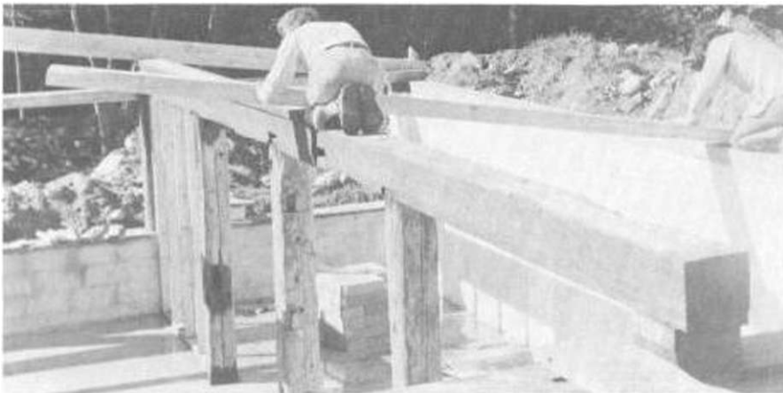
Illus. 7-7. The rafter is slid along the beams and put into position.
