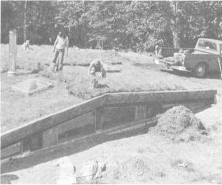
Illus. 112. Laying sod is easy: With the side of your foot, simply kick each new piece against those already laid.
