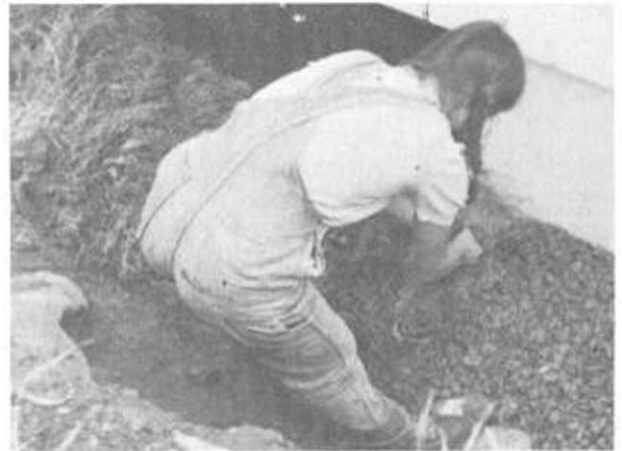
Illus. 10-5. Hay spread on top of the stones covering the footing drains will decompose and form a mat to stop infiltration into the drain by the subsequent sand backfill.
