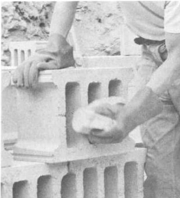
Illus. 6-1. Before slacking, a piece of broken block can be slid across other blocks to knock oil excess materials and burrs.
