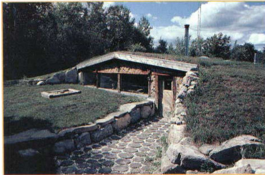
(Left) Log End Cave faces due south, West Chazy, N.Y. (Left, bottom) The stoves and stone mass at the center of Log End Cave (Below) North gable end of Log End Cave, with a stone circle made from boulders from the excavation
