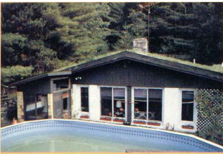
The Underground Studio, Jay, N.Y.
