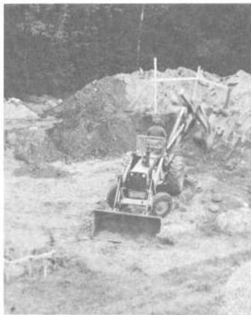
Illustrations 4-1 and 4-2. Excavating a hillside with a front-end loader and its 6'-bucket. The site should be excavated to a flat surface about 2' beyond the outside of the planned footing.
