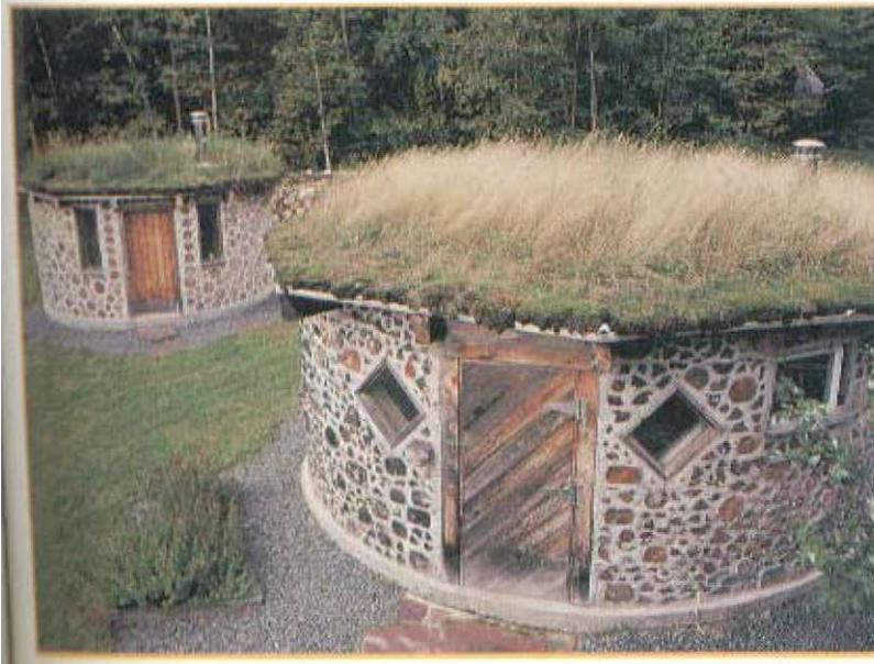
(Left, middle) Earthwood Building School, West Chazy, N.Y. (Left, bottom) Freestanding grass roofs on Earthwood outbuildings
