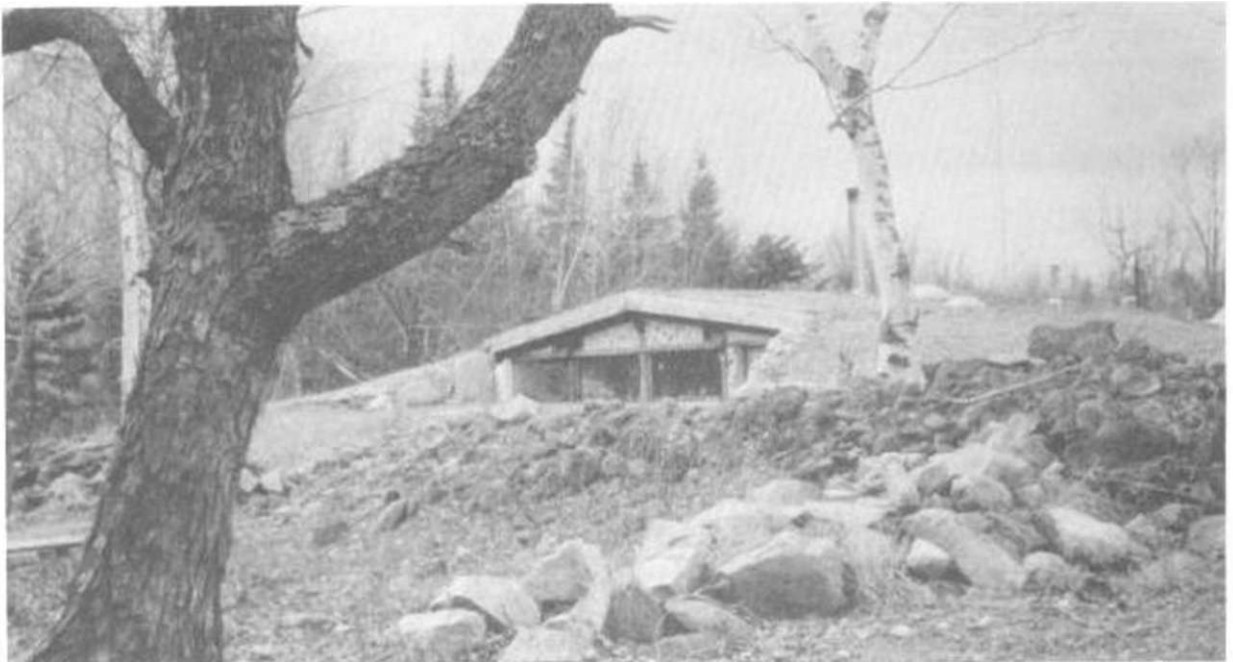
Illus. 13-3. The intent of the Log End Cave design was to have a minimal impact upon the landscape.
