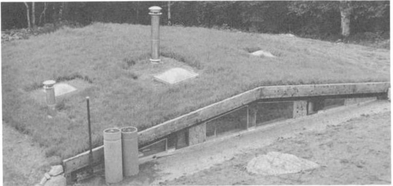
Illus. 13-4. The sod roof is in place. The north gnhlc windows admit light to the back rooms.
