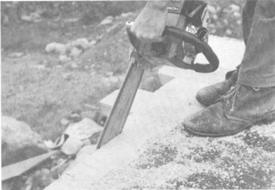
Illus. 8-6. Leave the plank ends sticking out. The overhang can be trimmed later by snapping a chalkline and cutting the whole edge at once.
