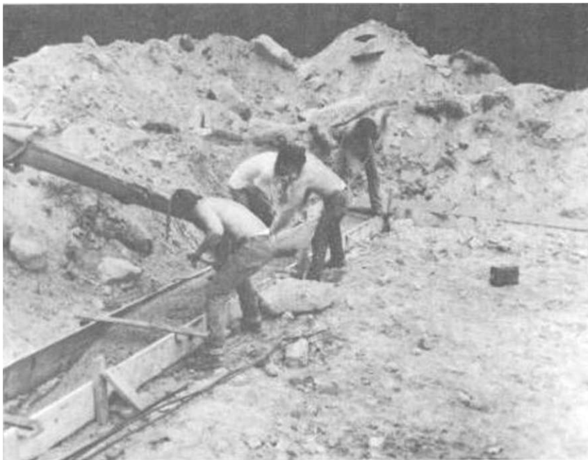
Illus. 4 11. A crew of four or five, each with a good strong rake, should be sufficient to draw the concrete around the footing ring.
