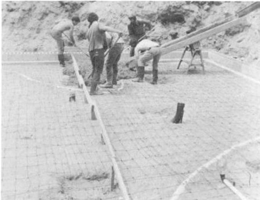
Illus. 5-10. Wire mesh holds the floor together if for any reason cracks develop in the concrete.
