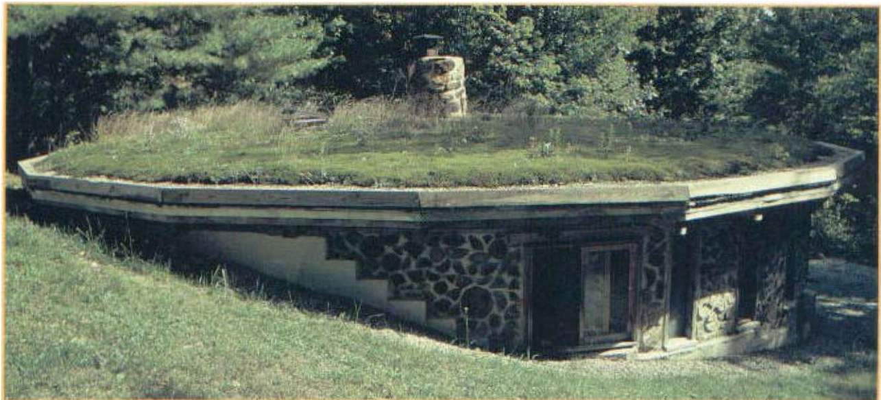
"Earthwood Junior," a single-storey version built by Paul Mikalauskas in Ashland, N.H. (Paul Mikalauskas photo)
