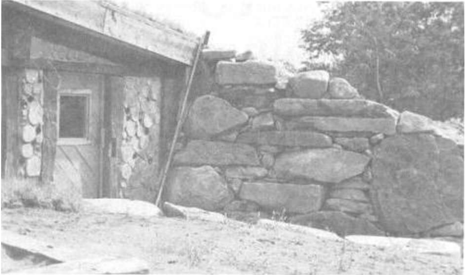
Illus. 13-1. The large triangular spaces left between the boulders can be tilled with smaller stones.
