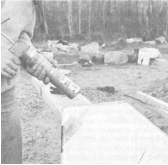
Illus. 12-2. Double-caulk the windows by running a bead of silicone along the glass itself and another bead along the molding surface to be placed against the sill or lintel.
