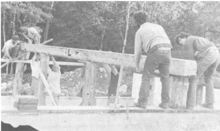
Illus. 7-4. The beam was then cantilevered over the north wall and positioned on the posts.
