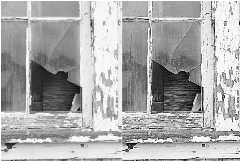
FIGURE 11-7 The image on the right shows the result of sharpening the details to accentuate the textural qualities.
