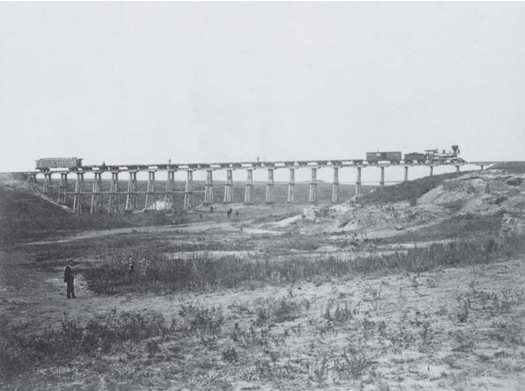
8.3 Alexander Gardner, View Near Fort Harker, Kansas, 216 Miles West of Missouri River; Across the Continent on the Kansas Pacific Railroad (Route of the 35th Parallel) , ca. 1867–68. Albumen print, 6 × 8 in. (15 × 20.3 cm.). Rochester, N.Y., George Eastman House.
