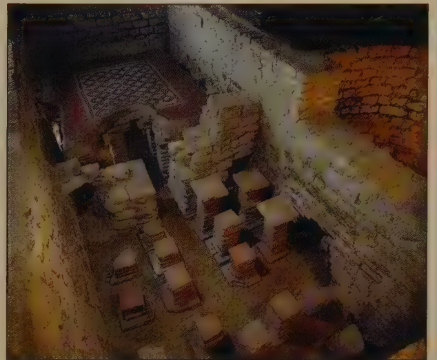
CHEDWORTH (Gloucestershire) (NT) Chedworth is the best surviving Roman villa in Britain. This general view of the west wing shows the mosaic floor of the warm room, the hypocaust pillars of the hot room and the semi-circular bath
