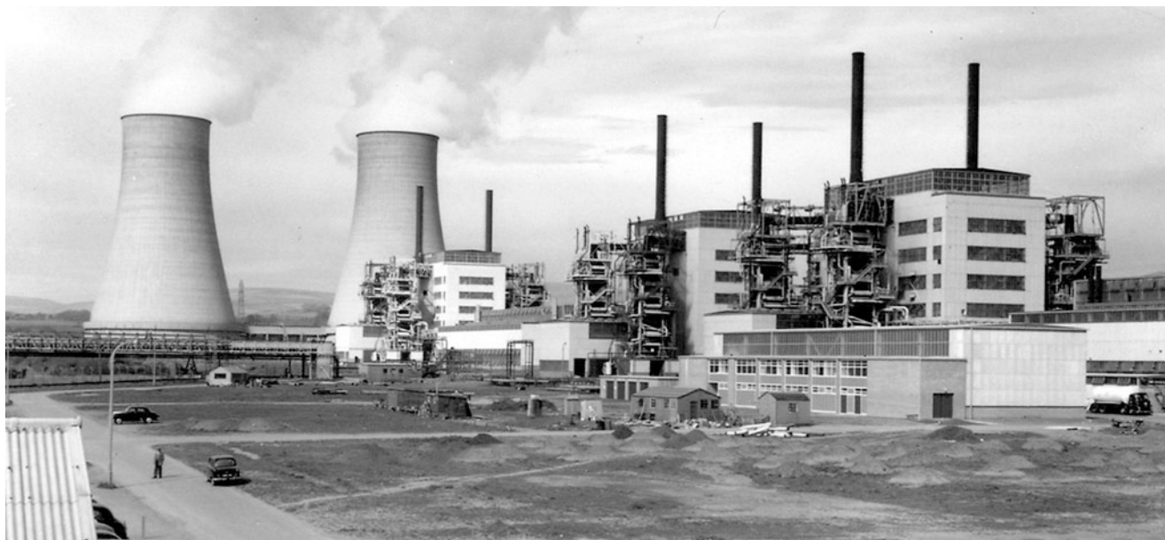
Fig. 27 Calder Hall, soon after opening, with its two reactors, two cooling towers, and turbine house. A further two reactors and two cooling towers were later added. Modern reactors generate far more power than Calder Hall. (Public sector information licensed under OGL v3.0)
