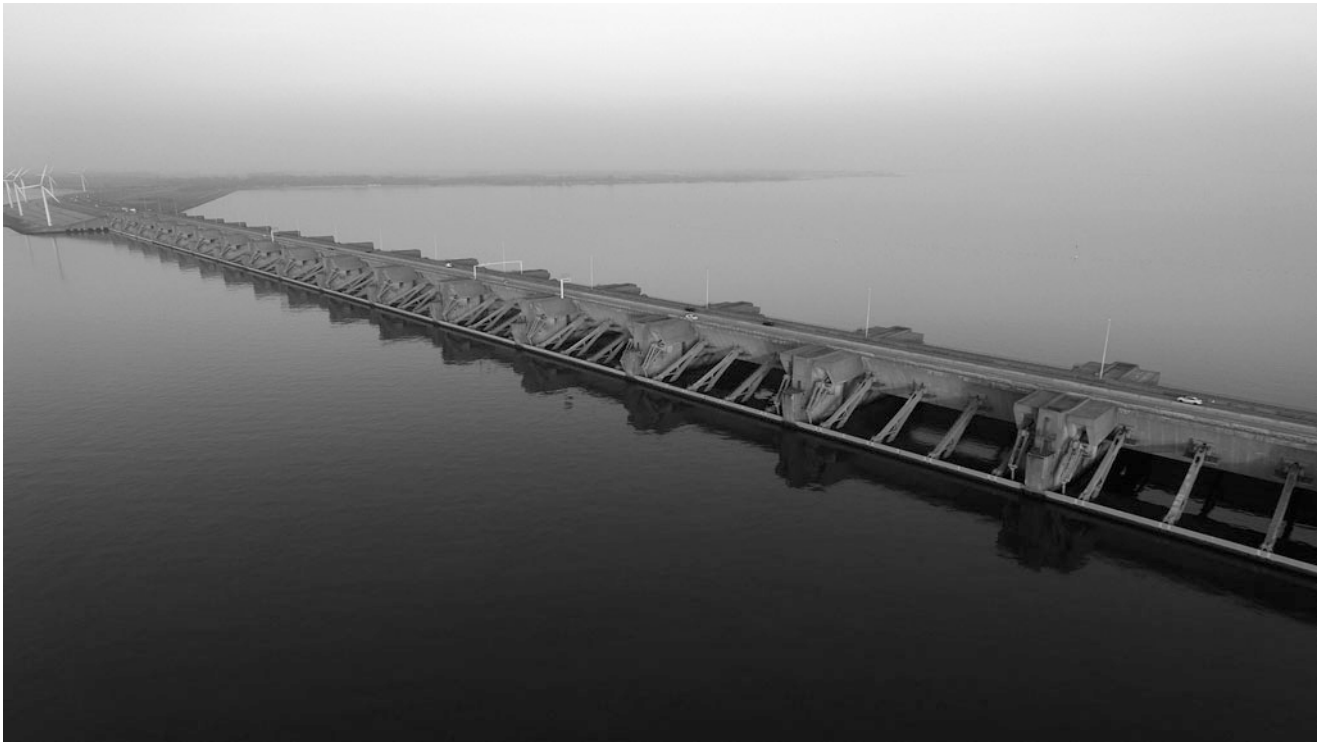
Fig. 29 The 5-km-long Haringvlietdam, which connects the islands of Voorne-Putten and Goeree-Overflakkee by road, is part of the Delta Works—a set of barrier protection works against the North Sea.
