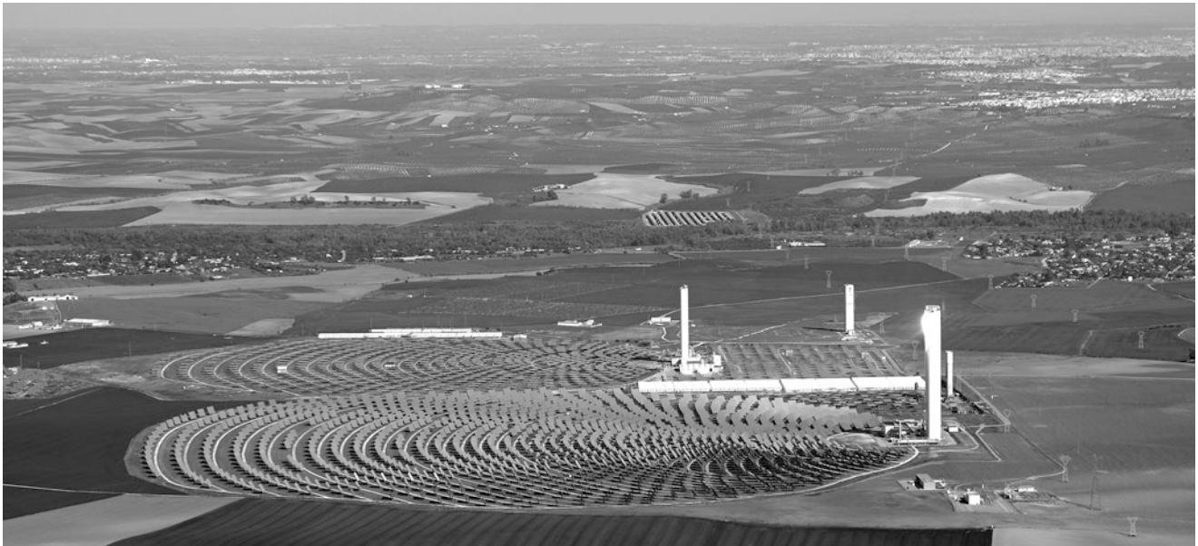
Fig. 26 In the decade 2010–2020, solar has steadily increased its share of renewable power generation. This image shows the PS20 solar power plant, which is part of the Solucar Complex in Seville, Spain. The PS20 has an array of large, moveable mirrors, called heliostats, that reflect sunlight to the top of a tower. The heat is used to turn water into steam,
