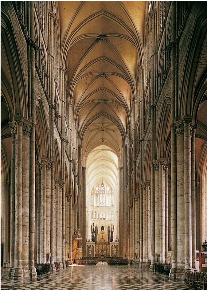
13-19 ROBERT DE LUZARCHES, THOMAS DE CORMONT, and RENAUD DE CORMONT, interior of Amiens Cathedral (looking east), Amiens, France, begun 1220.
