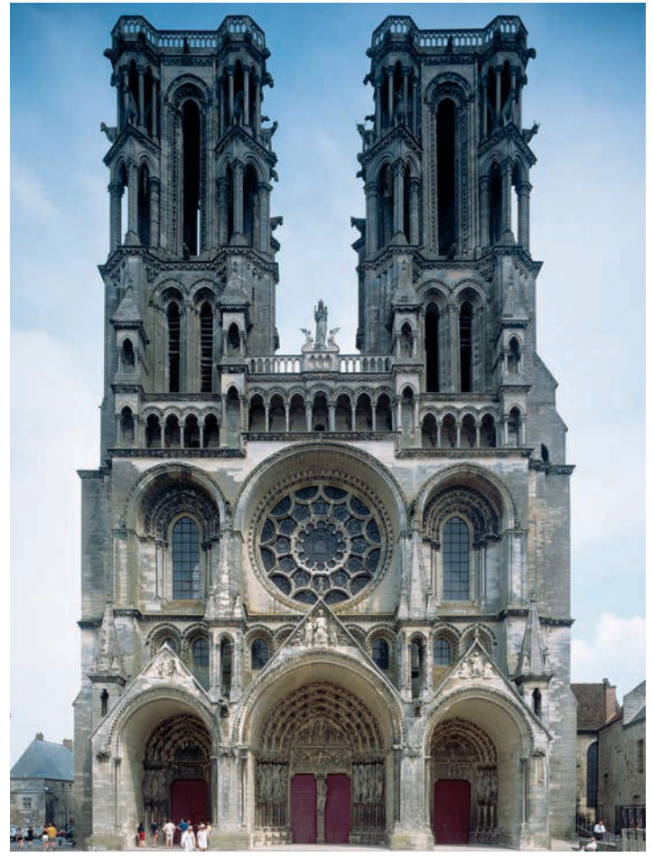
13-8 West facade of Laon Cathedral, Laon, France, begun ca. 1190.
