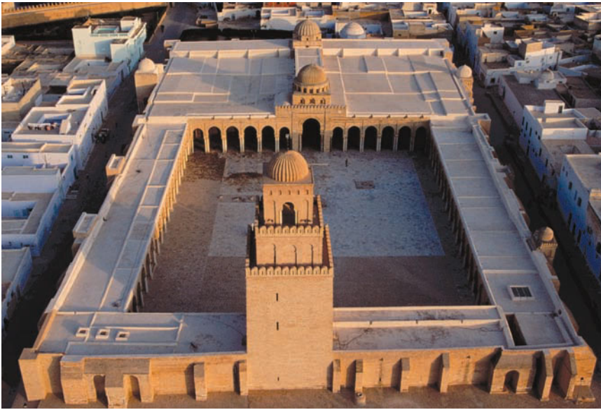
10-8 Aerial view ( left ) and plan ( right ) of the Great Mosque, Kairouan, Tunisia, ca. 836–875.
