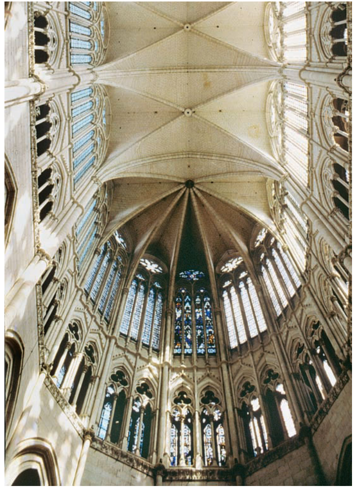
13-20 ROBERT DE LUZARCHES, THOMAS DE CORMONT, and RENAUD DE CORMONT, vaults, clerestory, and triforium of the choir of Amiens Cathedral, Amiens, France, begun 1220.
