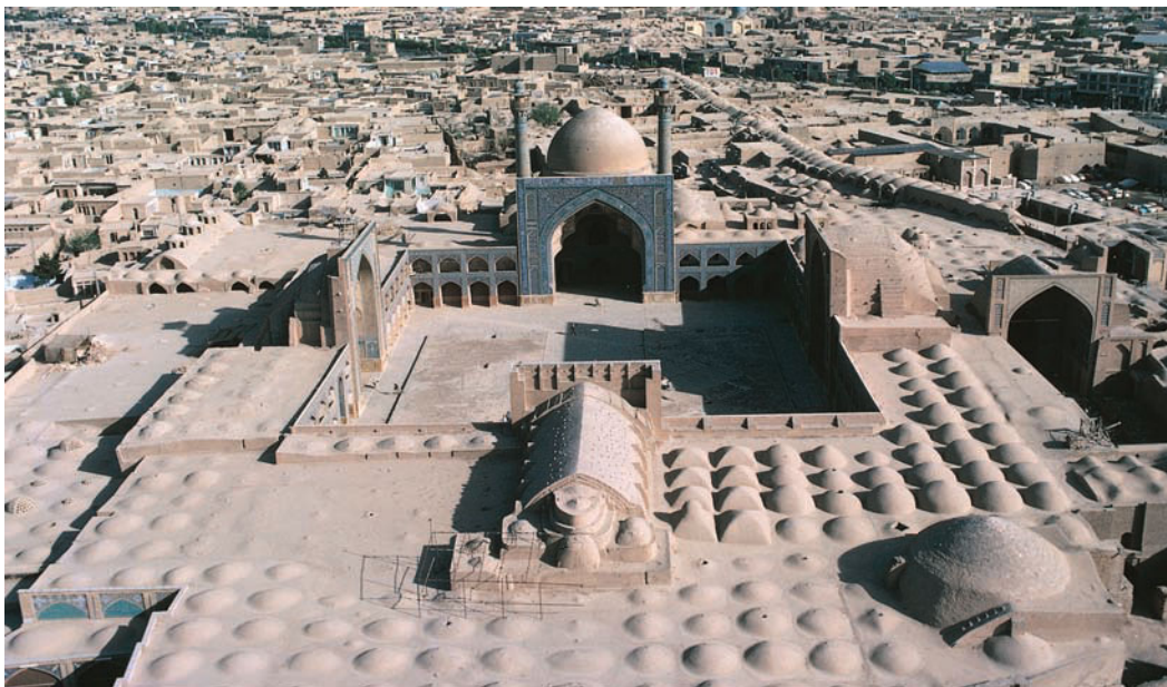
10-22 Aerial view (looking southwest) of the Great Mosque, Isfahan, Iran, 11th to 17th centuries.
