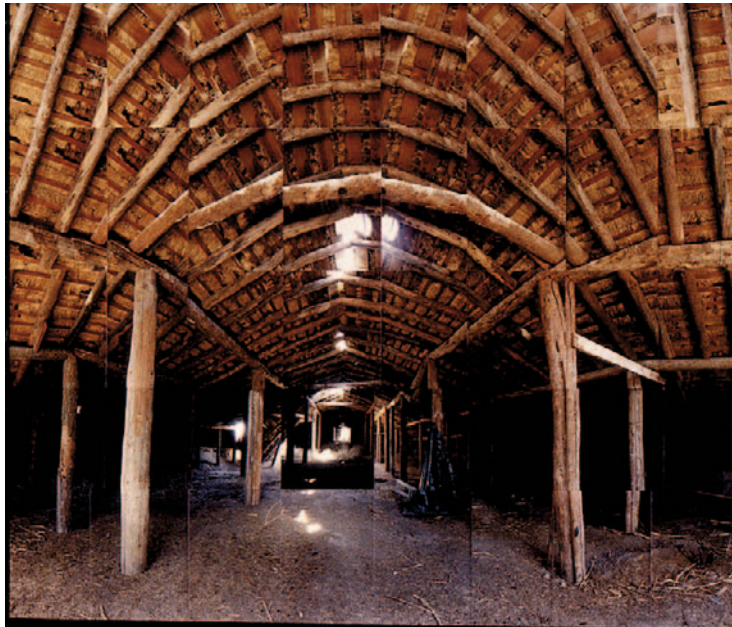
Figure 15.10 Joiners are not intended as accurate depictions of space. If you want to make the joins invisible then you can do this digitally. This image, created using multiple photographs, by Masumi Hayashi is of the Minidoka Relocation Camp, Root Cellar 1992 (one of the relocation camps used to house the Japanese in the USA during WWII). Hayashi used joiner image techniques for her series American Relocation Camps to explore her own personal relationship to the spaces where she had been interned as a child with her family
