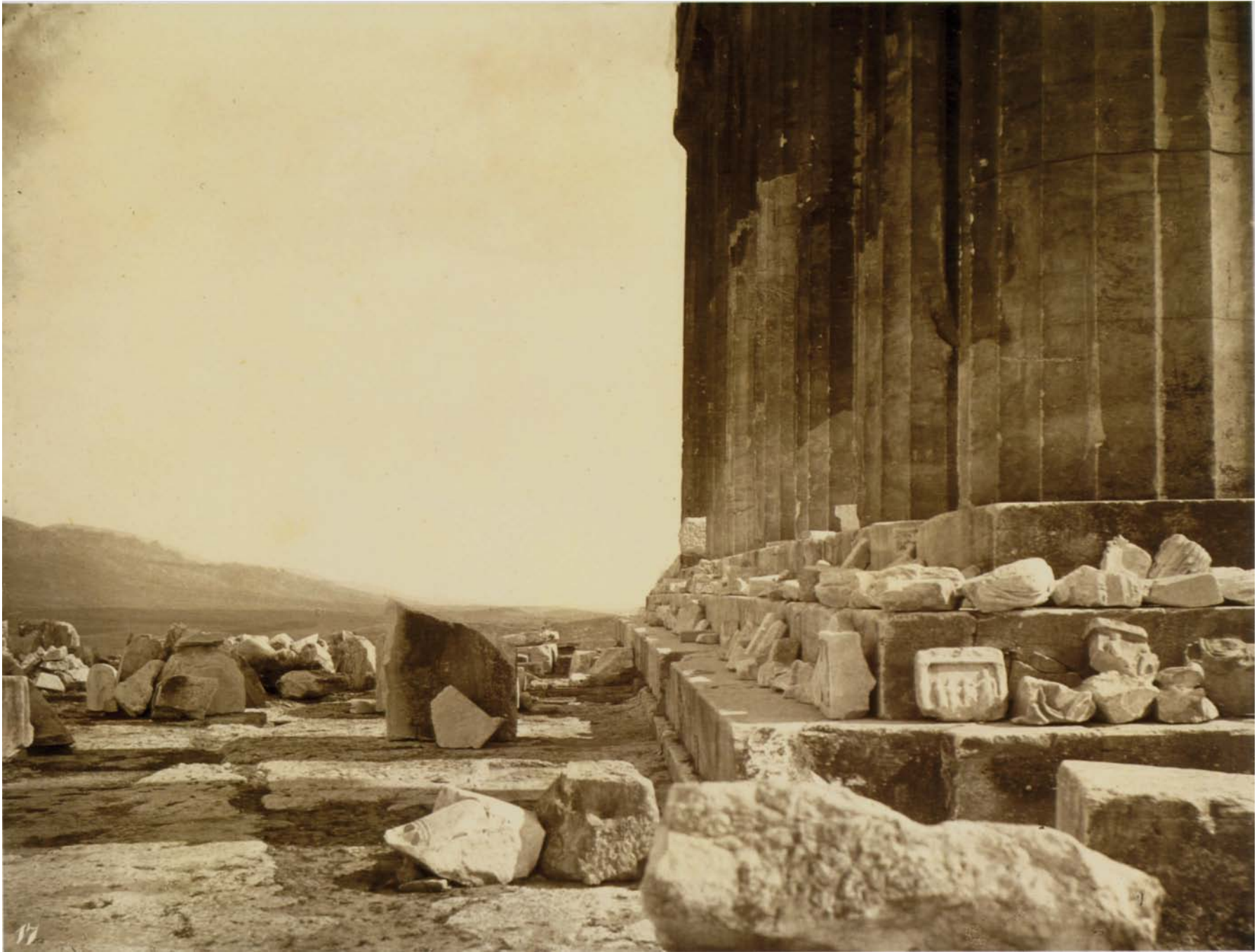
Figure 15. WILLIAM JAMES STILLMAN (American, 1828–1901), Profile of the eastern façade [of the Parthenon], showing the curvature of the stylobate, 1869. From The Acropolis of Athens (1870), Plate 17. Carbon print, 18.4 × 23.8 cm (7¼ × 9⅜ in.). JPM 84.XO.766.4.18.
