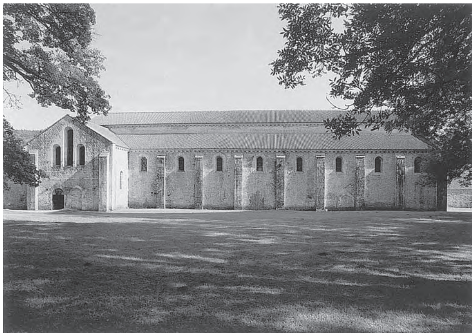
FIGURE 27-4 Fontenay (Côte d’Or), France. Fontenay illustrates the modest scaled overall form, with square-ended terminations, a low presbytery, and a tower-less crossing and window-less barrel vaulted nave associated with the “Bernardine” church.
