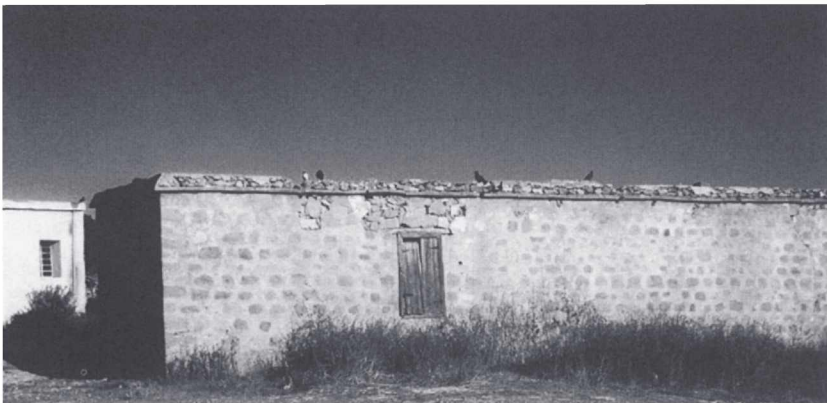
Plate 5. An abandoned village house
