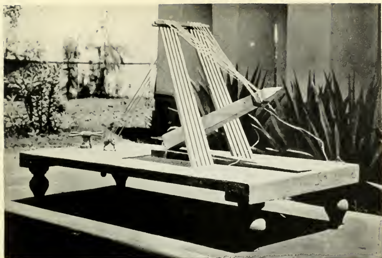
FIG. 41. MODEL SHOWING HOW THE PARIS OBELISK WAS LOWERED AND ERECTED. (Page 116.)
