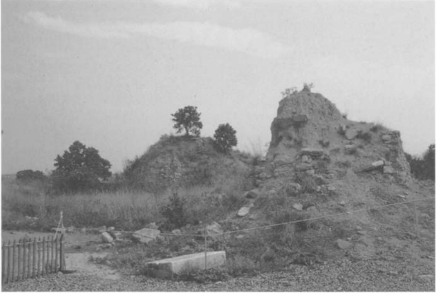
8 The construction site: Troy in 1989.
