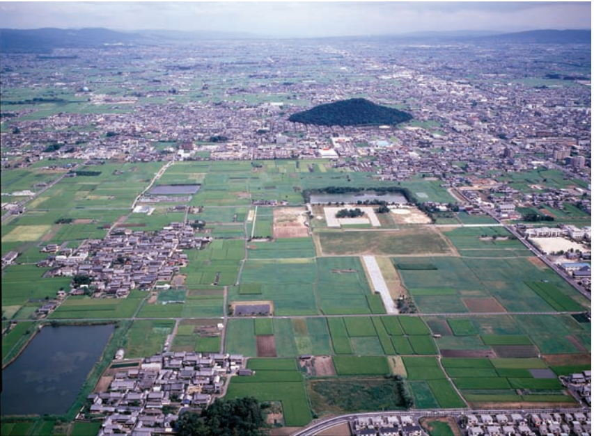
Fujiwara Palace site. Facing north toward Miminashi yama; archeological site of palace with Daigokuden in the center. Source: Nara bunkazai kenkyūjo sōritsu gojū shūnen kinen. Asuka, Fujiwara-kyō ten , 137.
