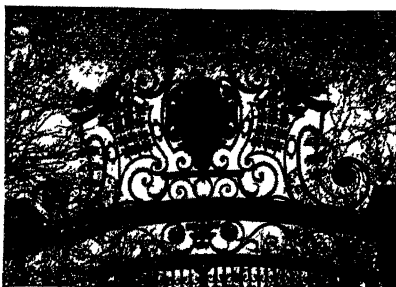
6 Ironwork, Gate of House at Aix
