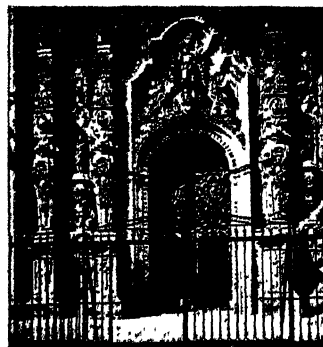
5. DETAIL, FACADE of SAGRARIO MEXICO CITY
