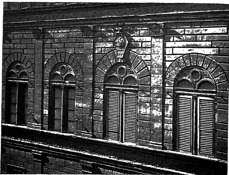
FIGURE 26. DETAIL, FAÇADE OF PALAZZO RUCELLAI, FLORENCE.
