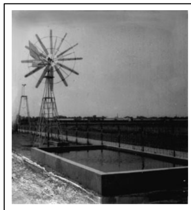
Fig. 13.14 A typical windmill installation for irrigation. Note the water storage tank in the foreground
