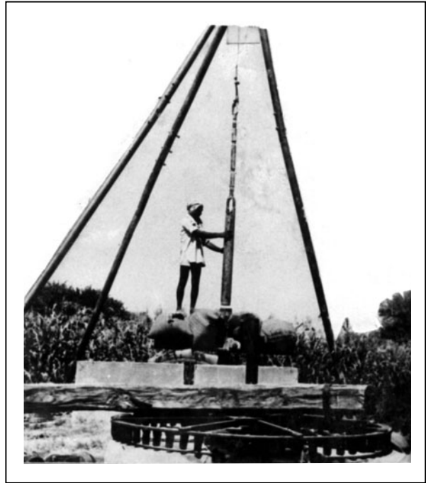
Fig. 3.12 Boring in an open well. Note the cutter bailer ready to be inserted into the casing pipe. The cog wheel in the foreground is the drive wheel of a Persian wheel installed in the well
