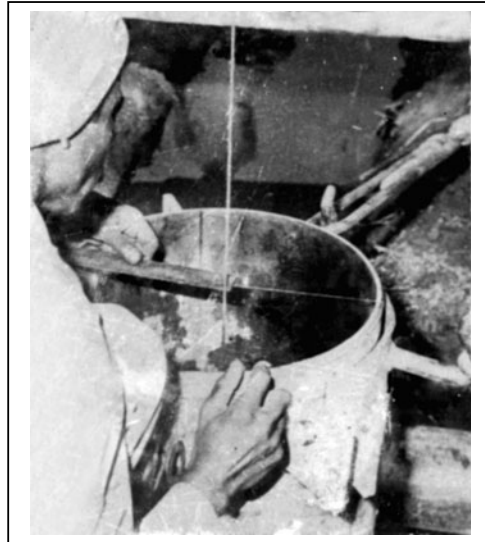
Fig. 5.62 Measurement of deviation of plumb line from the centre of a tube well at its top
