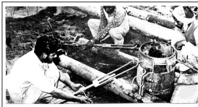
Fig. 5.63 Procedure for straightening a tube well. Note the plumb line, cross wires and jacks
