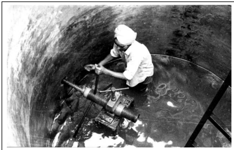
Fig. 3.23(b) Radial boring equipment in operation in an open well
