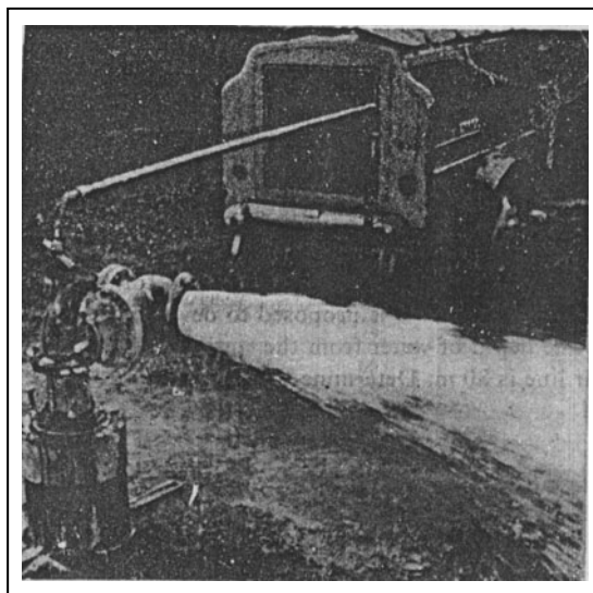
Fig. 6.7 Tube well development with compressed air
