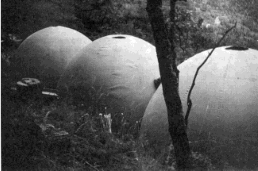
Rear view of the domes, covered by the air forms
