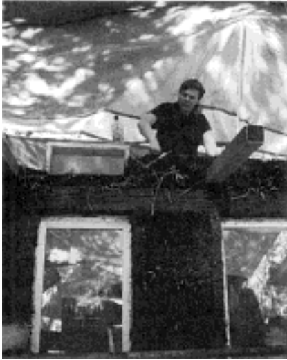
Nearing the top of the wall
