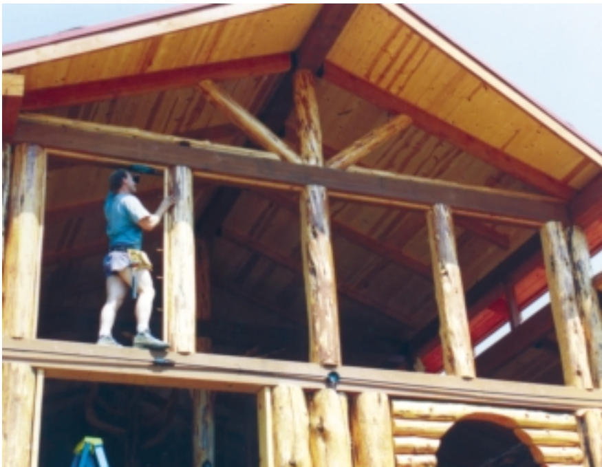
Kirt installs picture window stops with screws.
