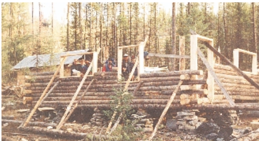
The walls go up.
