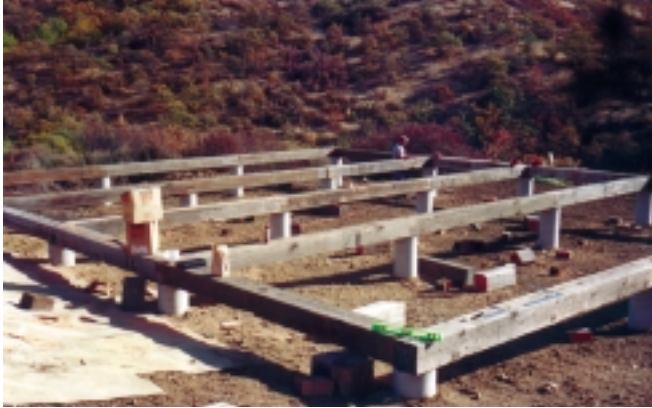
Kirt works on foundation grid.
