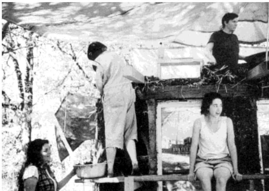
Supports for this scaffolding are built into the wall. When the project is finished, they'll simply be sawed off.
