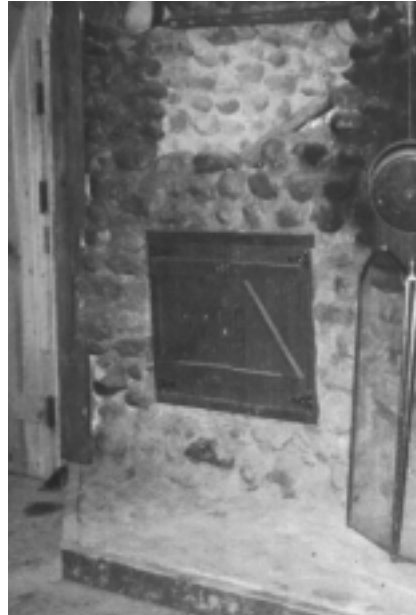
The interior doors of our through-the-wall woodbox are located right next to our big fieldstone fireplace, allowing us to fuel the fireplace with ease. The design illustrated below is different from this one.
