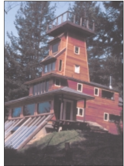
Figure 4: (Below) A water tower can be converted into a house.
