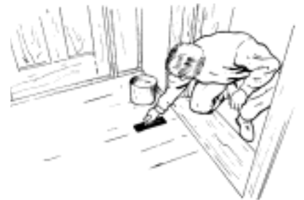
Fig. 9. Apply the leveling compound with a trowel.
