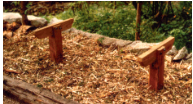
Bench posts set into place awaiting the seat
