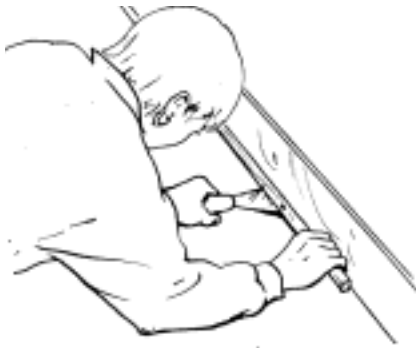
Fig. 2. Remove baseboard quarter-round moulding or vinyl wall base with a tool such as a putty knife.
