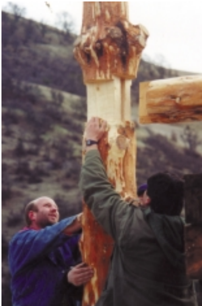
Eric, Dorothy's son (left), Vadim, and Kirt guide the horizontal beam with tenon into its mortise on the upright log.
