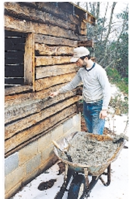
The walls when chinking began. Notice how large the spaces were.
