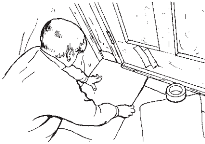
Fig. 5. Tucking the pieces of felt under the threshold.
