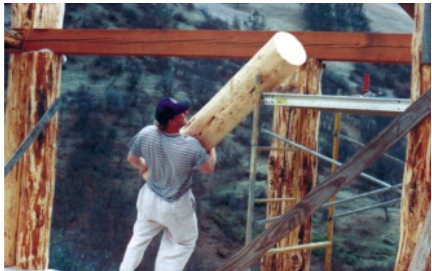
Kirt hefts the ridgepole supports onto the scaffolding.
