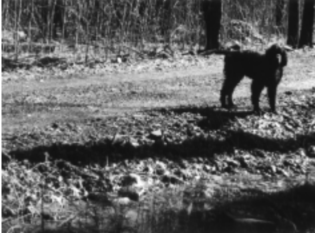
This picture illustrates the height of the road, which is 4 to 6-feet deep in places.
