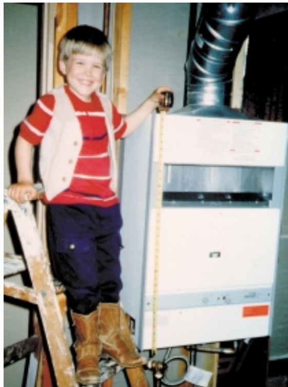
Is your hot water heater smaller than a four-year-old? Benjamin Guiltner shows how this Aquastar measures up. The model shown in the photo is one of the largest tankless heaters available.
