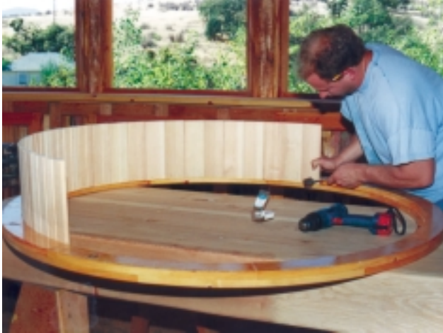
Kirt builds the round window for living room.
