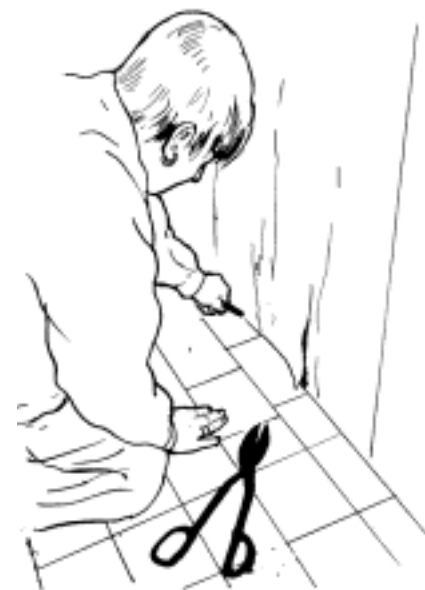
Fig.13 Use a crayon to mark the edges that need trimming.
