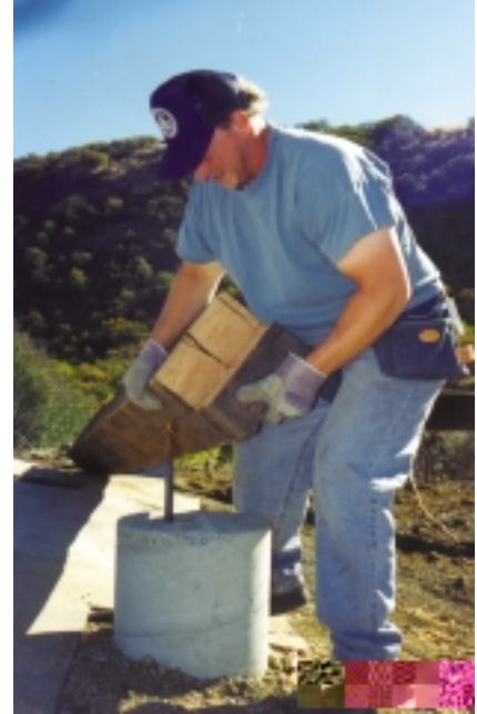
Kirt places foundation beam.
