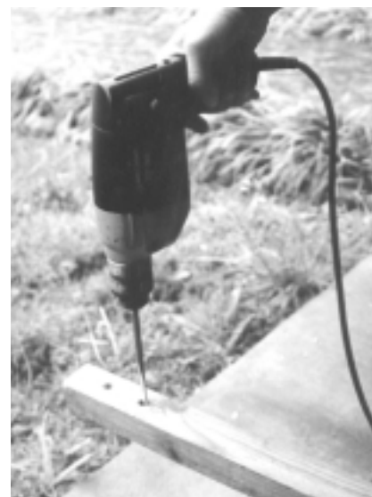
Drilling the holes for the extension pole
