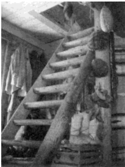
A stairway made from logs, using a chain saw, hammer, and chisel. The steps are set into the split log.
