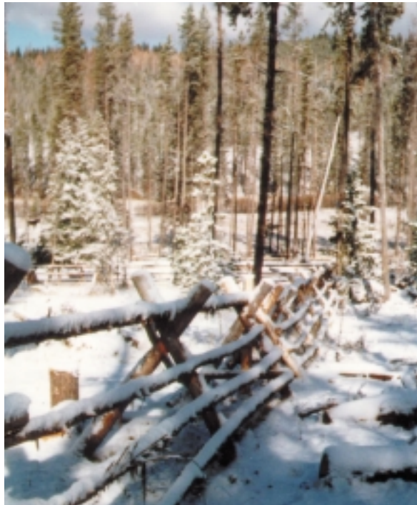
A jackleg fence made from dead lodgepole pines.
