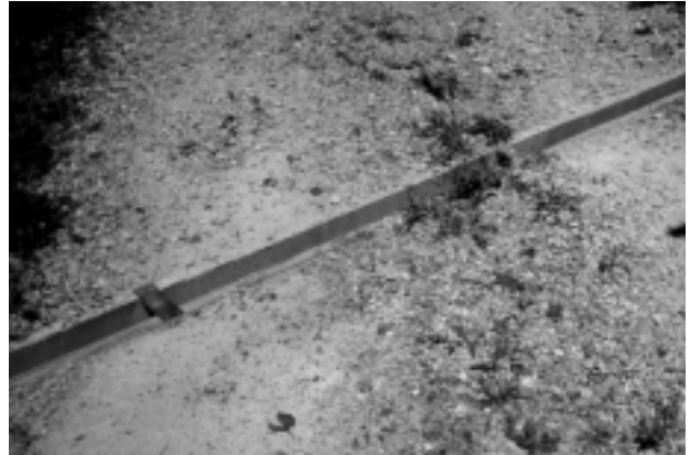
The water break crosses the road at an angle.
