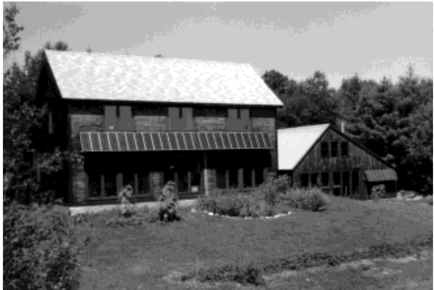
The Fowlers' home has solar modules on the house and on the garage.
