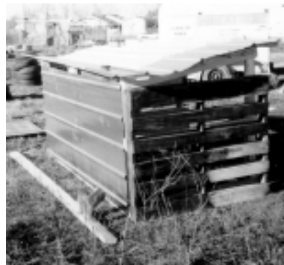
Figure 2. A pallet is used for the end of the shed and there is another in the middle which divides the shed into two individual stalls. Metal sheeting is used for the roof, the back, and the end of the shed that faces the wind.
