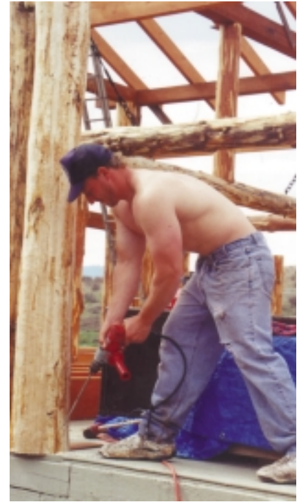
Kirt predrills log. He will toenail it to the deck with 12-inch polebarn spikes.
