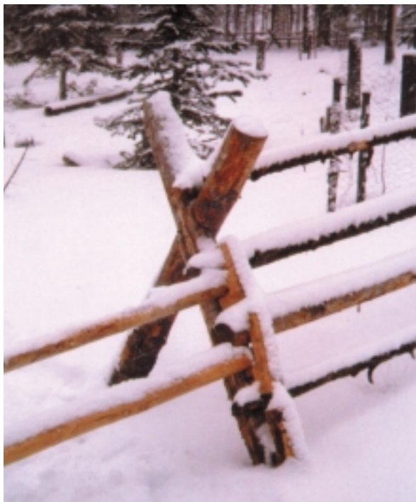
Detail of the construction of a jackleg fence.
