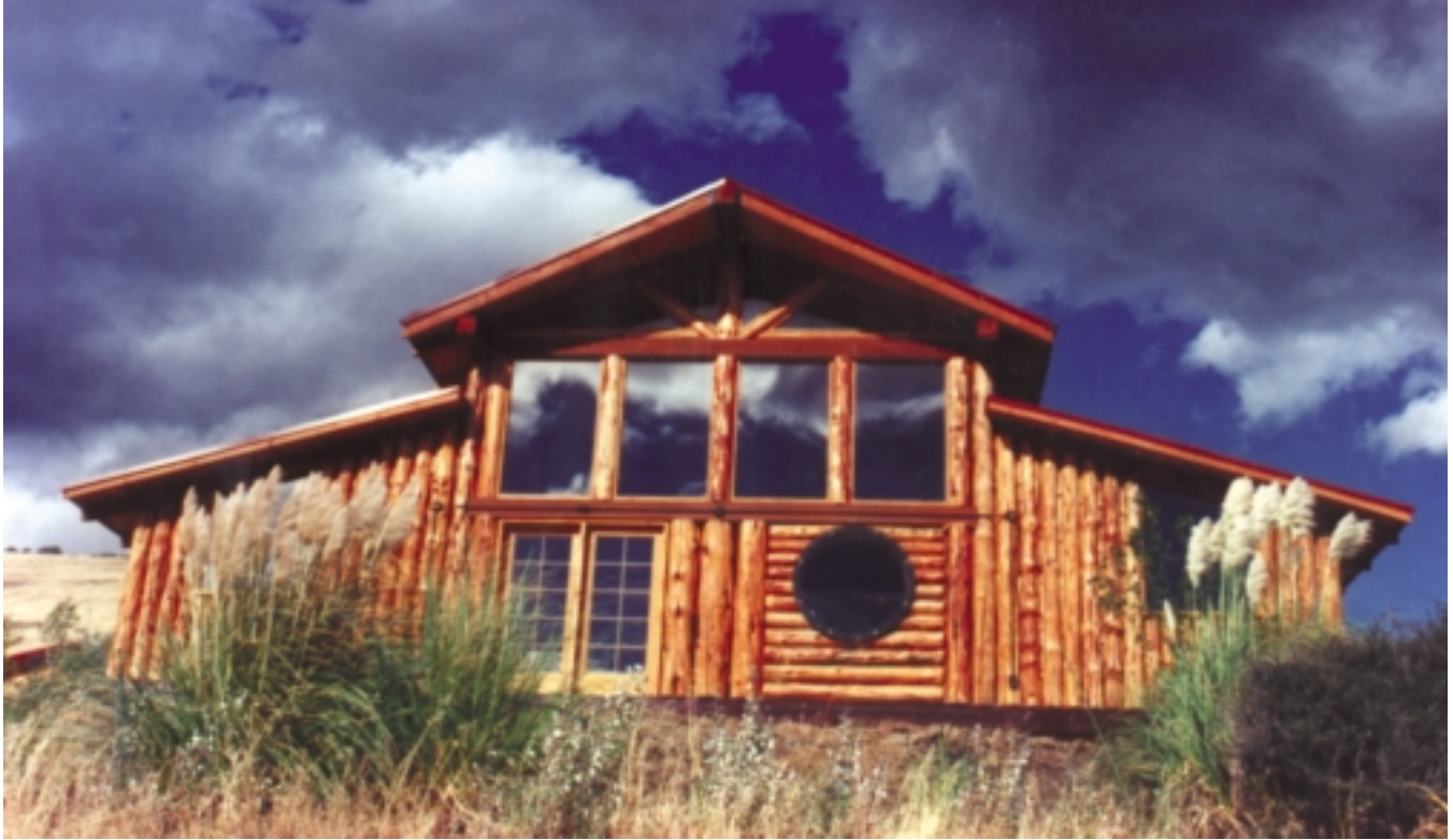
The completed second log home
