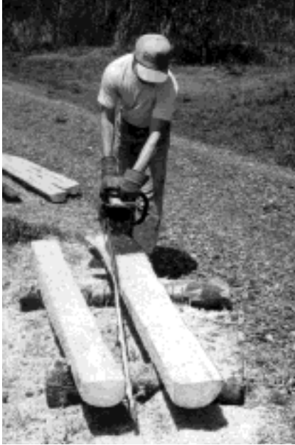
We lay the halves smooth side up and then trim off the edges. Smooth edges make the planing much easier.
