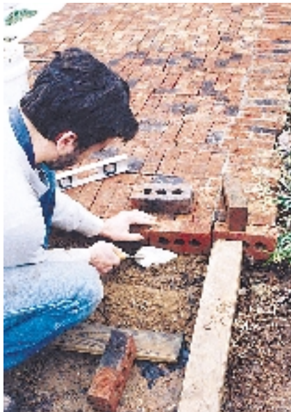
Figure 1. Use a trowel to smooth the sand for the next bricks.
