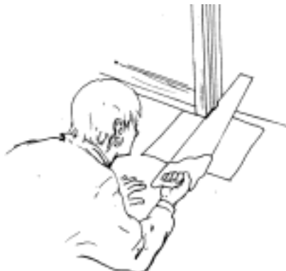
Fig. 3. Cut out the bottom of the door mouldings with a carpenter's hand saw held flat, right at floor level.
