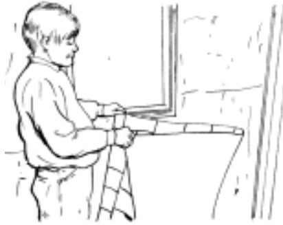
Fig. 14. The correct method to lift the flooring, to apply the adhesive, while being careful to avoid damaging it.
