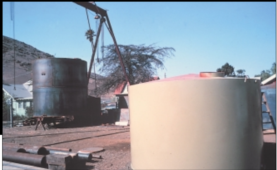
Figure 1: Welded tanks are transported to the storage site.
