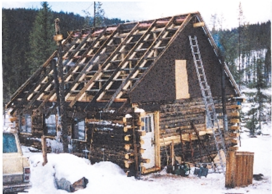
The log home before the roof went on.
