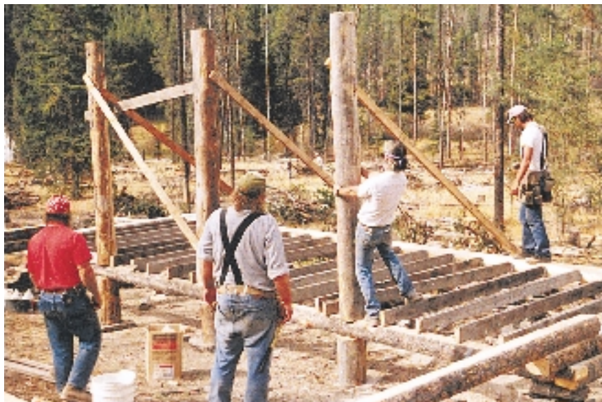
The beginning of the construction of Dynah's log home.
