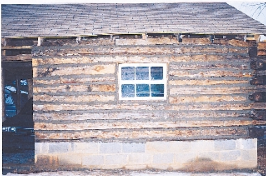
The building when the chinking was completed.
