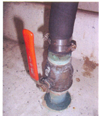
Through Hull Fitting
