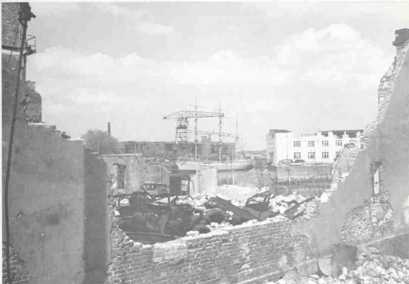
A blasted-out window frames Horst Wessel during her fitting out to become Eagle, amid the ruins of Bremerhaven and its Weser River harbor, during the hard and unsure spring of 1946. (U.S. Coast Guard Archives photo)
