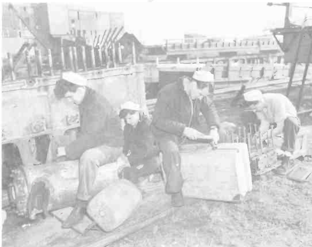
Coast Guardsmen wrestle with bits of pieces of the ship's M.A.N. diesel engine under arduous post-war conditions. A stroke of good fortune and English good will provided a usable replacement block, but the entire engine remained in use until its replacement in 1982. (U.S. Coast Guard Archives photo)
