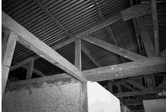
Figure 9: Careful jointing between columns and beams improves structural integrity ©Practical Action /Chris Martin
