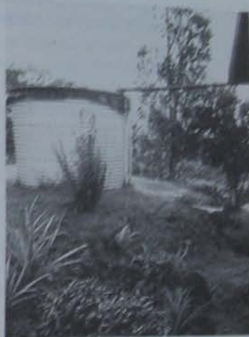
Rainwater harvesting provides all domestic water by gravity for a house near Hilo, HI.
