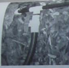
Flexible PVC is a work- ing tinkertoys set for moving water or waste water without glue (or leaks) at pressures up to 10 psi.
