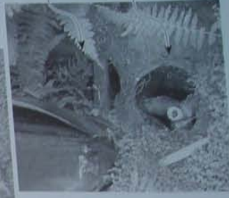
Outlet chamber Greywater splitter access chamber
