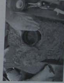
Making a lid, access port: Cut out a section between structural ribs with a sawsall or keyhole saw.
