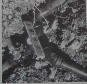
Subassembly is then glued into the system as a unit.
