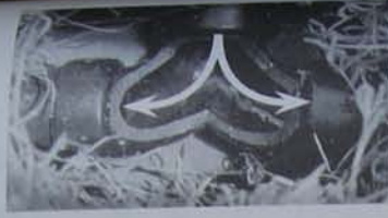
Cutaway view of a double ell, a flow-splitting fitting that is largely self-cleaning with no filtration. This one is part of the first known Branched Drain network. I valiantly tried to clog it with pure kitchen sink water—took the sink strainer out and pushed bowls of scrag granola and pot scraps down the pipe for half a year. The p-trap clogged every other day, but the Branched Drain network never did.
