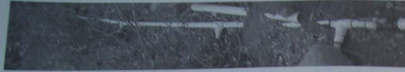
An exception: "Twisted Tees" system in Santa Fe, NM has been successfully tuned so that the same amount of laundry water comes out each outlet, which branch off progressively lower until the end.
