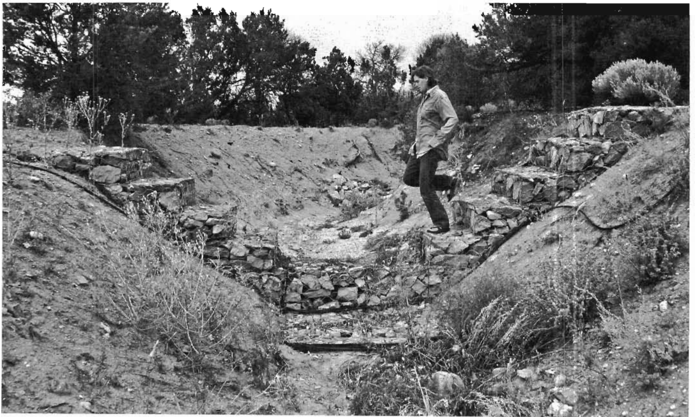
Fig. 10.23. Gabion steps crossing a drainage. Work by Santa Fe Permaculture
