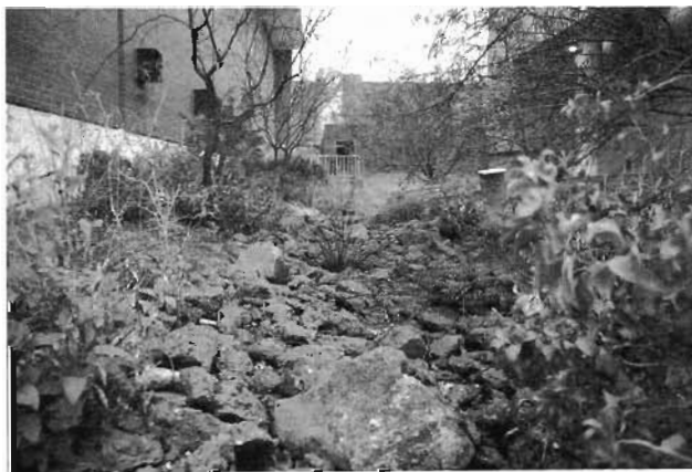
Fig. 7.16B. After - porous cobble infiltrationway after the concrete was jackhammered and left in place. The infiltrating water passively irrigates the native vegetation growing through the cobble. For color photo see inside back cover.
