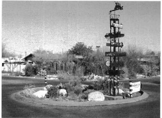
Fig. 8.5C. New traffic circle with raised curb, but no curb cuts. Used where center of road or intersection is raised or crowned to drain water to side of road. Raised curb (and sunken, mulched basin within) retain rainfall that would otherwise run off. Note: The construction of this circle reduced the paved area of the intersection by 26%!
