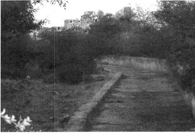
Fig. 9.10A. A stabilized diversion swale built to collect hillside runoff and redirect it to a cistern in the Jaipur Fort built in 1726, Jaipur, India. This diversion swale and the cistern are still in use. The Maharaja opened the fort to the public in 1983, and it is now a tourist attraction.
