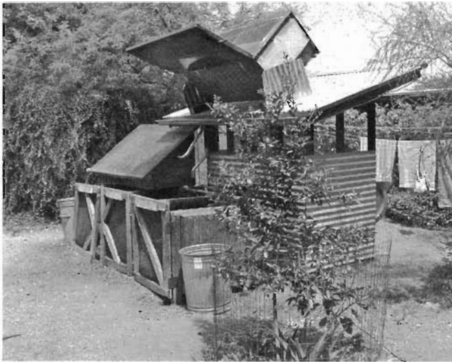
Fig. 12.28A. Wash and Well, front view. The batch-style solar water heater on compost bins heats water for the outdoor shower behind the vine-covered wall. The solar water heater atop the laundry shed roof is for the washing machine. An old refrigerator is used for the heater's insulated box. Its door can be closed to hold in more heat at night, and then opened again in the morning to let in the sun.
