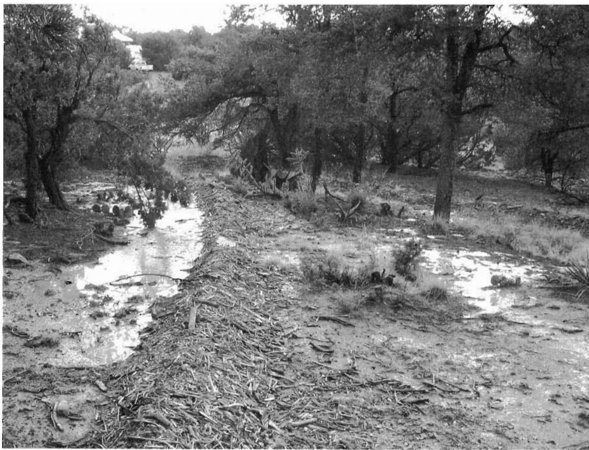
Fig. 7.14. Contour berms of woodchips. Chris Meuli's land, Edgewood, New Mexico. Credit: Chris Meuli
