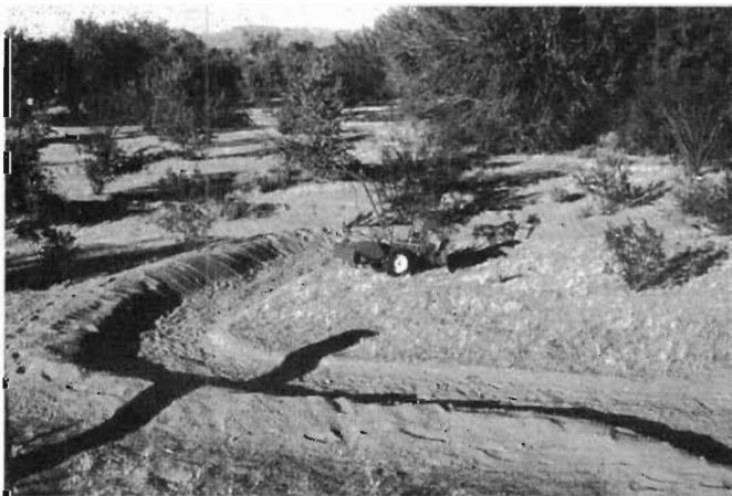
Fig. 2.11. Contour berm dug with rototiller, with dirt from basin becoming the downslope berm. Credit: Tim Murphy
