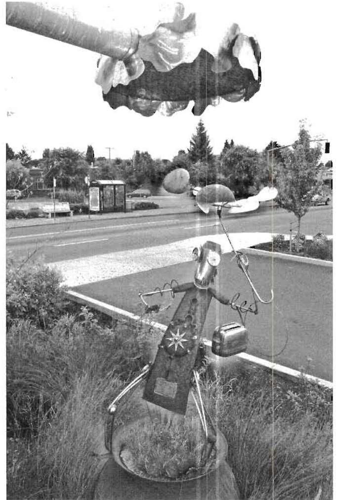
5.30. Celebrate the rain! Roof runoff from the New Seasons Market showers down from a cloudlike downspout onto a sculpted figure within a rain garden. As the falling water hits and moves the figure's propeller umbrella, the figure also starts to move and dance in the rain. Portland, Oregon
