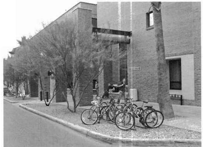
Fig. 8.15B. Porous aggregate under bike racks and trees in heavy pedestrian zone, University of Arizona, Tucson. Runoff from concrete sidewalk is harvested in porous aggregate, while sidewalk and curb help keep aggregate in place. Trees would benefit even more if the section of impervious concrete between pillars and palm tree were replaced with an extension of pervious pavement.
