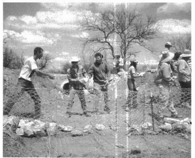
Fig. 10.19. Bucket-brigade rock delivery
