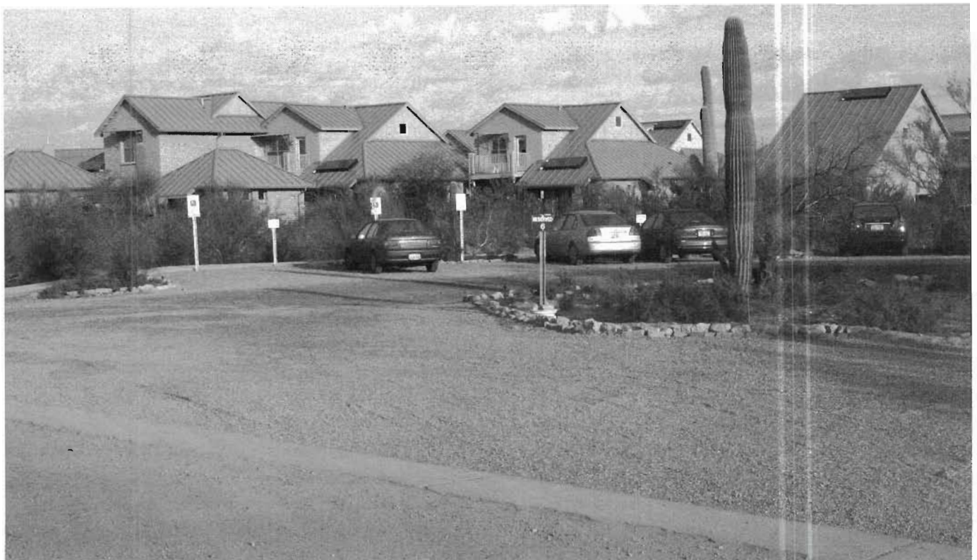
Fig. 8.17B. Completed Gravelpave 2 parking lot with geocells filled with gravel. There is no runoff from this parking lot, so no detention basin or other drainage infrastructure was required. See the first Real Life Example in chapter 5 and figure 5.23 of the Milagro plan for more.
