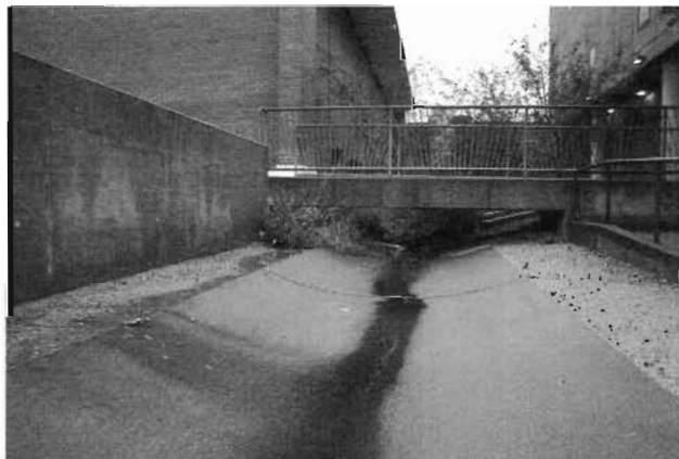
Fig. 7.16A. Before - impervious concrete drainageway . South of Architecture building, University of Arizona, Tucson, AZ. For color photo see inside back cover.
