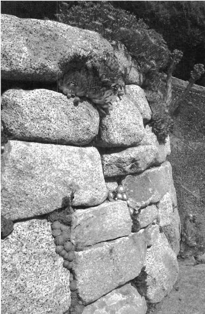
Fig. 3.15. Vegetation between retaining-wall rocks. Stonework by Goettling McGee, Inc., Seattle, Washington.
