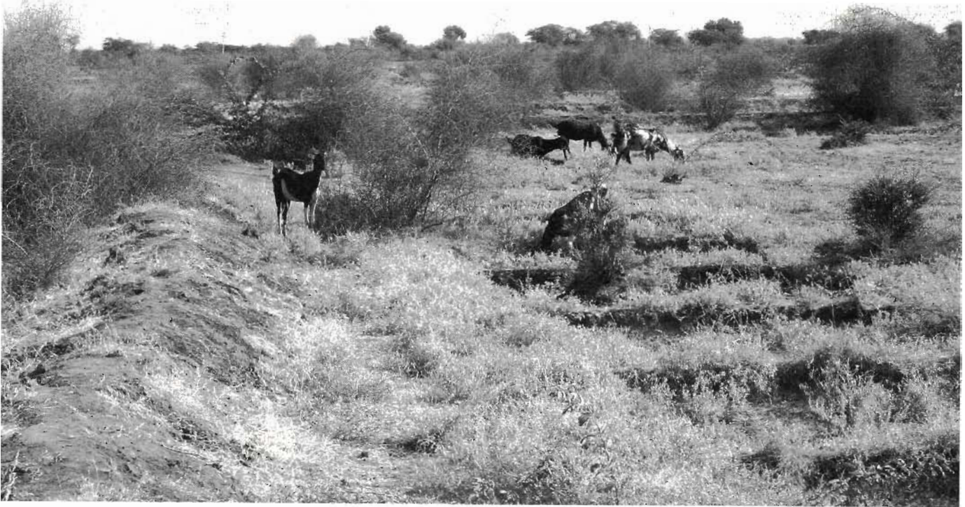
Fig. I.17. Goats browsing in pasture of choukas in the neighboring village of Sahalsagar. Runoff flows in from right side of photo. Chouka berm on left stops the runoff and spreads the water back over the pasture to the right. The square basins upslope of the berm were dug out to obtain soil for the berm.
