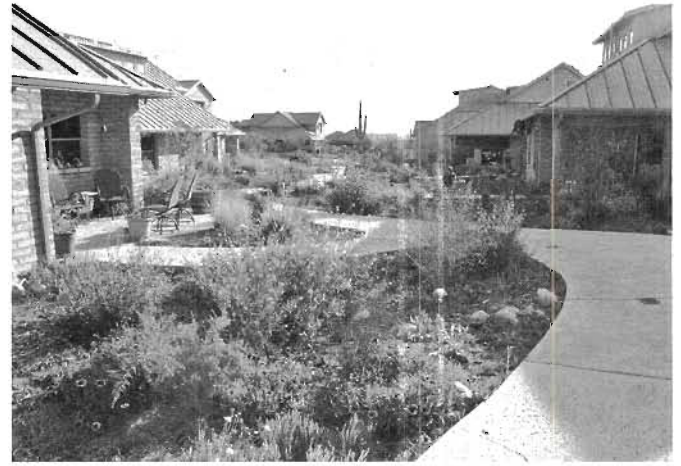
Fig. 5.24B. Same basins mulched and vegetated. Basins are designed to infiltrate water quickly so there are no problems with mosquitoes or anaerobic soils. These basins, with their spongy mulch and soil-burrowing plant roots, infiltrate all water within 20 minutes.
