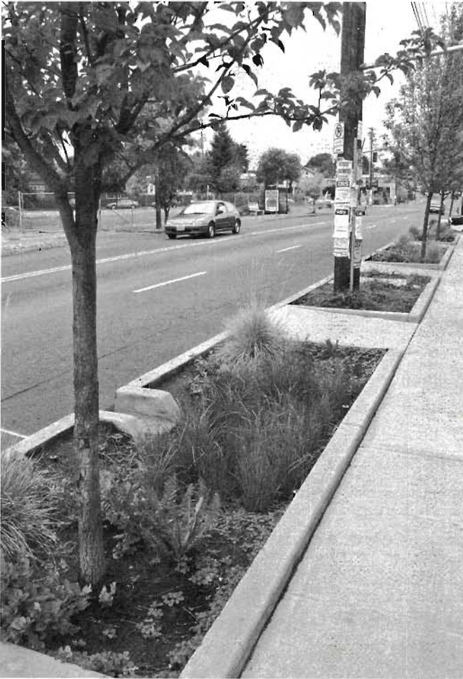
Fig. 8.28. Curb cuts along an arterial street beside the New Seasons Market direct runoff into adjoining mulched and vegetated basins. Portland, Oregon
