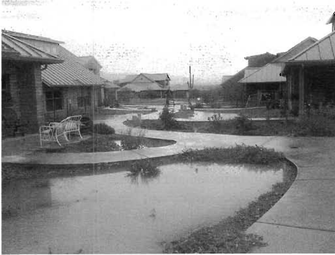
Fig. 5.24A. Rainfall collected in newly constructed infiltration basins minutes after a large summer storm. The basins have not yet been mulched or planted. Milagro Cohousing, Tucson, Arizona. Credit: Natalie Hill.
