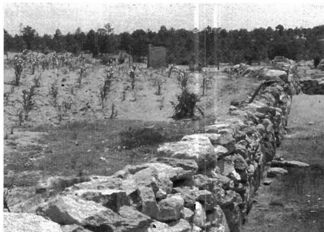
Fig. 3.18. New trinchera and field at Rowerachi, Chihuahua, Mexico in 2002. Note the batter or lean of the wall into the slope. Credit: Barney Burns.
