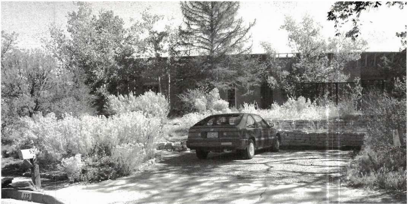
Fig. 4.12. The driveway has been cut down to the length of a car and the width of two. It is paved with porous open-graded aggregate, and sloped toward the base of the terrace retaining wall where a French drain infiltrates any runoff. The terraces, rain- and greywater-irrigated vegetation, and metal trellis help screen out headlights at night. Ben Haggard residence, Santa Fe, New Mexico
