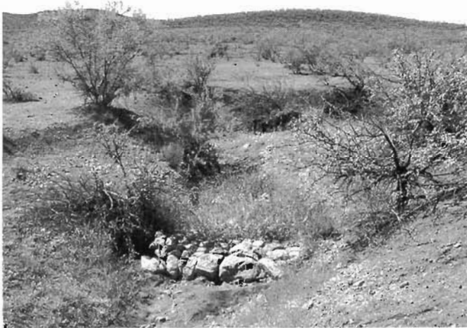
Fig. 10.29B. Two months later, after summer rains, new vegetation has grown upstream of the stabilizing dam. Reproduced with permission from An Introduction to Erosion Control by Bill Zeedyk and Jan-Willem Jansens. Photo credit: Van Clothier
