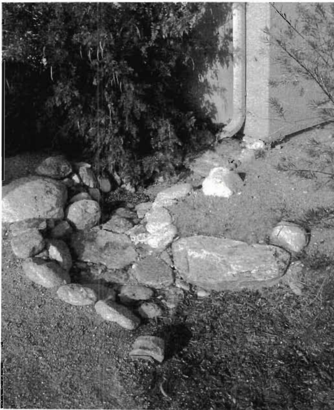
Fig. 5.18B. Stone-stabilized downspout spillway
