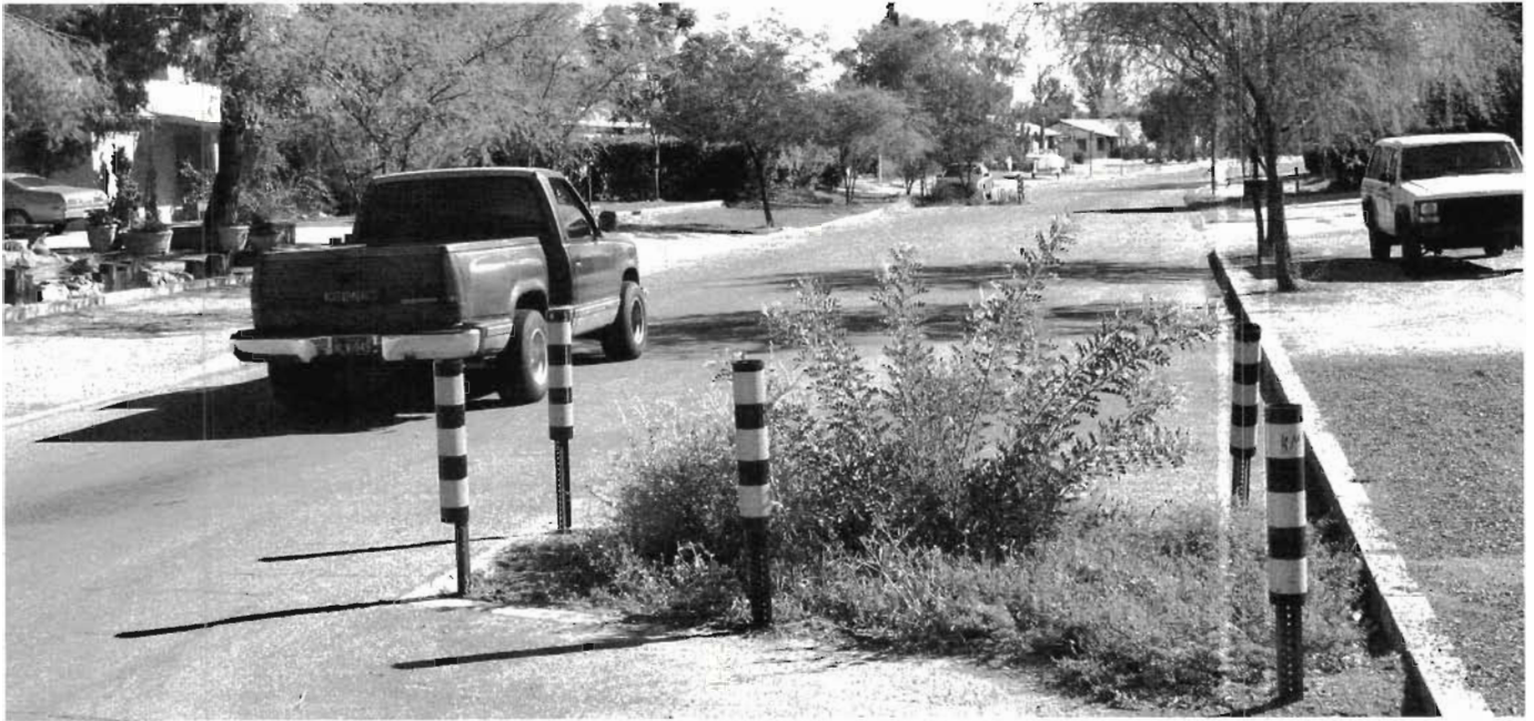
Fig. 8.6. Chicanes or pullouts with flush curbs. Used where road is crowned or raised in the center and drains runoff to streetside curb. Flush curb allows runoff to infiltrate soil of planting area, while surplus runoff can continue down the street. These pullouts calm traffic by forcing it to meander. Speed humps in the area constricted by pullouts could calm traffic even more if needed.
