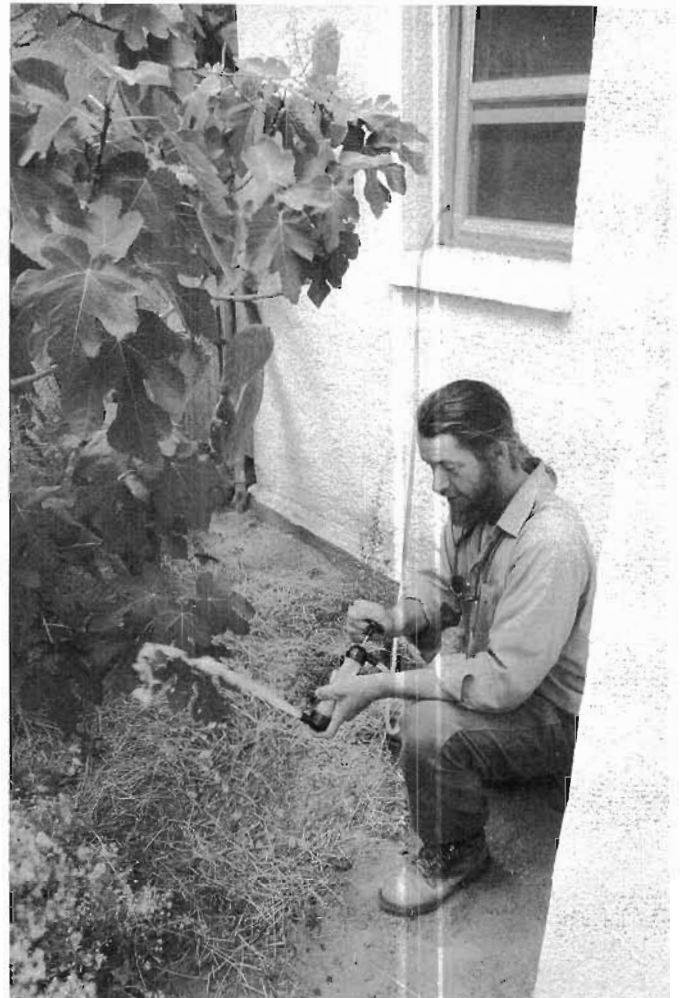
Fig. 12.16B. Exterior siphon hand pump (from auto parts store) pulls tub greywater through tube. Once water is flowing, the pump is pulled off, the tube is placed in a mulched basin with fig tree, and the siphon effect continues to draw the water. Purchase the hand pump first so you can select the correct tube diameter to fit the pump.
