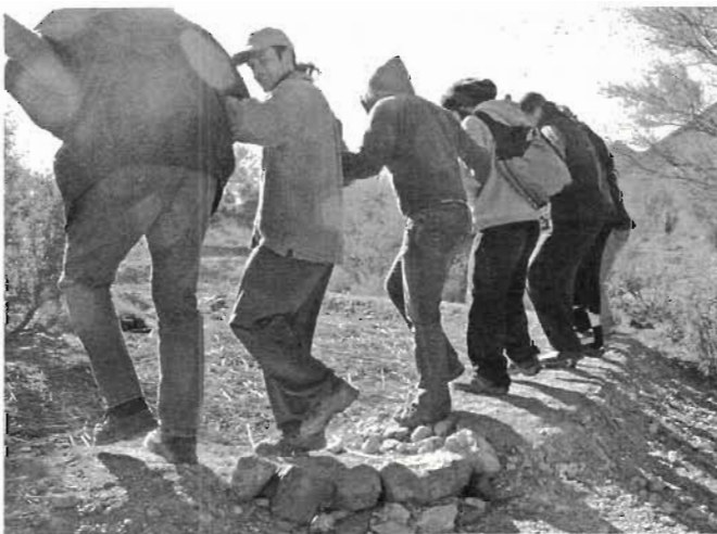
Fig. 2.15. A line of folks stomping/tamping the berm with their feet
