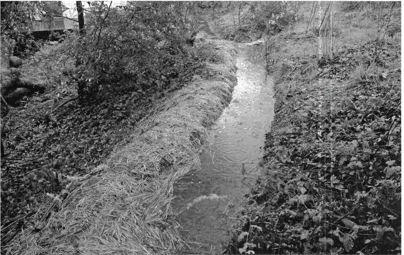
Fig. 11.8. A section of a 60-foot (18-m)-long, 2.5-foot (0.75-m)-wide, 1.5-foot (0.45-m)-deep, two-tiered berm 'n basin full of rain at Occidental Arts and Ecology Center in northern California. In 2006, 96 inches (2,438 mm) of rain fell, resulting in this b'n'b harvesting over 600,000 gallons (2,274,000 liters) of runoff. Most of the water comes from a 4-inch (100-mm)-diameter drainpipe from a diversion drain installed upslope to dewater a 1/3-acre (0.13-ha) area above a septic leach field. This pipe used to daylight onto a forested slope forming a gully 5 feet (1.5m) wide and 4 feet (1.2 m) deep, from which erosive sediment flowed down to contaminate a stream of spawning salmon. Now the gully has been stabilized, and the b'n'b intercepts the runoff to help recharge groundwater while improving the stream's water quality for the salmon. Such b'n'bs, typically with smaller catchments, are also used on the site to passively irrigate apple, apricot, peach, and plum trees. The trees are planted beside, but not within, the basins, so the root crown is better drained in this wetter climate. Credit: Brock Dolman.
