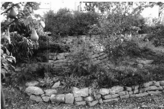
Fig. 3.1. Terraces stabilized with dry-laid walls made from salvaged concrete sidewalk or “urbanite” in the sloped backyard of the Zemach residence, Los Alamos, New Mexico
