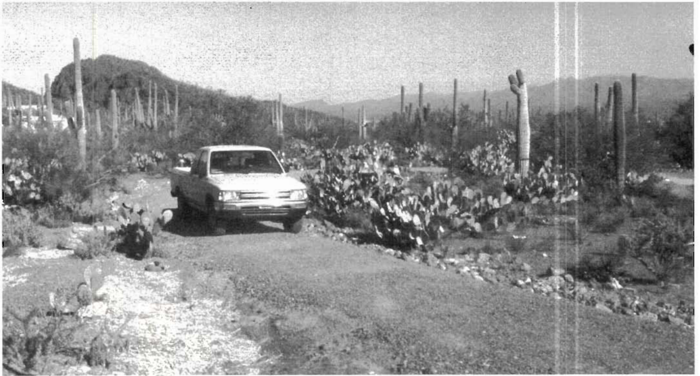
Fig. 2.25B. A berm as a raised driveway/road, Dancing Rocks Permaculture Community, Tucson, Arizona. The driveway runs along the contour, halting runoff from the land upslope. Mulched basins along the road then infiltrate the water to establish and enhance soil-stabilizing vegetation. The road surface is stabilized with stone and gravel collected on site when four building pads were excavated. The banks of the raised driveway could be further stabilized with larger rock if the need arises. Note that the driveway was kept as narrow as possible to reduce the negative impact to the landscape.
