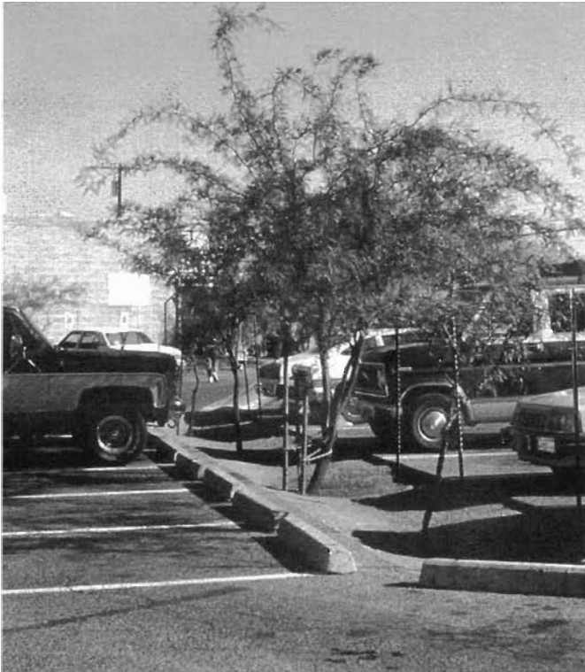
Fig. 8.11. Shade trees planted in a basin cut on contour in a once-solid asphalt parking lot. A bunyip water level was used to find the contour, and spray paint marked it before cutting. Parking bay strips were repainted to align with the basin. The speed hump (at the far end of the basin) acts as a diversion berm directing additional runoff into the basin. After one year, the trees could survive entirely on runoff from the building and remaining asphalt. This photo was taken three years after the trees were planted. Old Community Food Bank site, Tucson, Arizona. Note: Mulch would further enhance the water infiltration and storage capacity of the basin. Photo and design credit: Dan Dorsey
