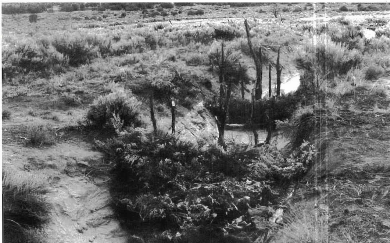
Figure 10.31. Brush check dams with punjie posts immediately upstream in the lower part of the Lallo arroyo on the Zuni Indian Reservation, Arizona. Note the waterlines behind the structures and the effect of brush clearing along banks. Reproduced with permission from “Native American Methods for Conservation and Restoration of Semiarid Ephemeral Streams.” Credit: Jay Norton
