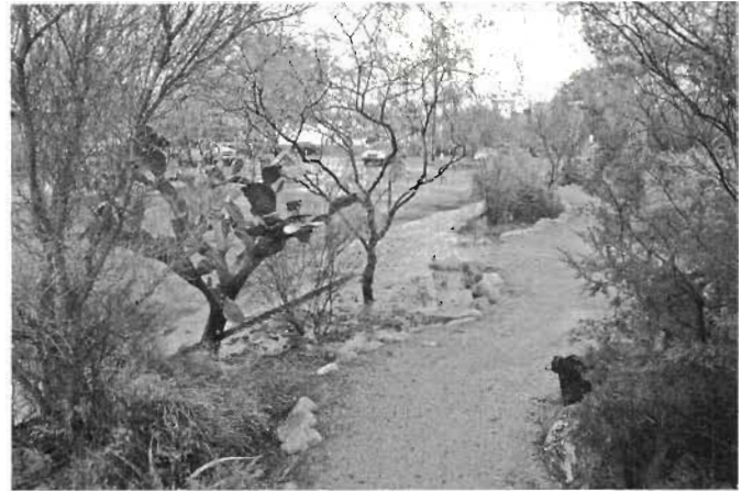
Fig. 5.12. Space was tight along this public right-of-way, so the resulting steep-sided edge between path and basin was stabilized and delineated with rock. Mulch and vegetation within the basins further discourage folks from stepping off the path. Note: Basin to left is low enough to capture street runoff, while higher basin to the right harvests runoff from the path.
