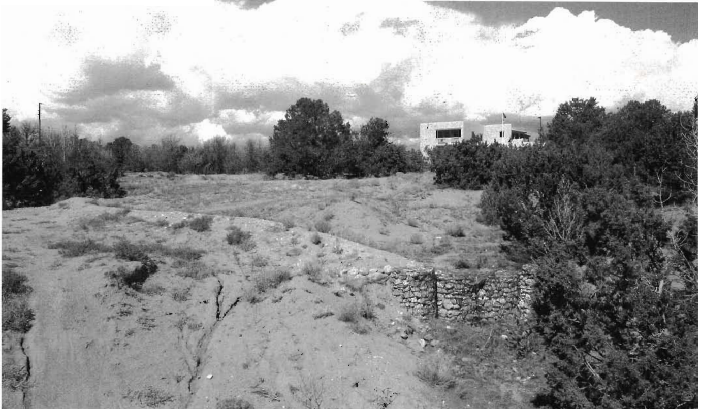
Fig. 9.9. An earthen diversion swale redirecting runoff away from an eroding steep slope, to a drainageway stabilized with a gabion. Note: A series of contour berms were first placed upslope of the diversion swale to start harvesting water at the top of the watershed. Santa Fe, New Mexico.
