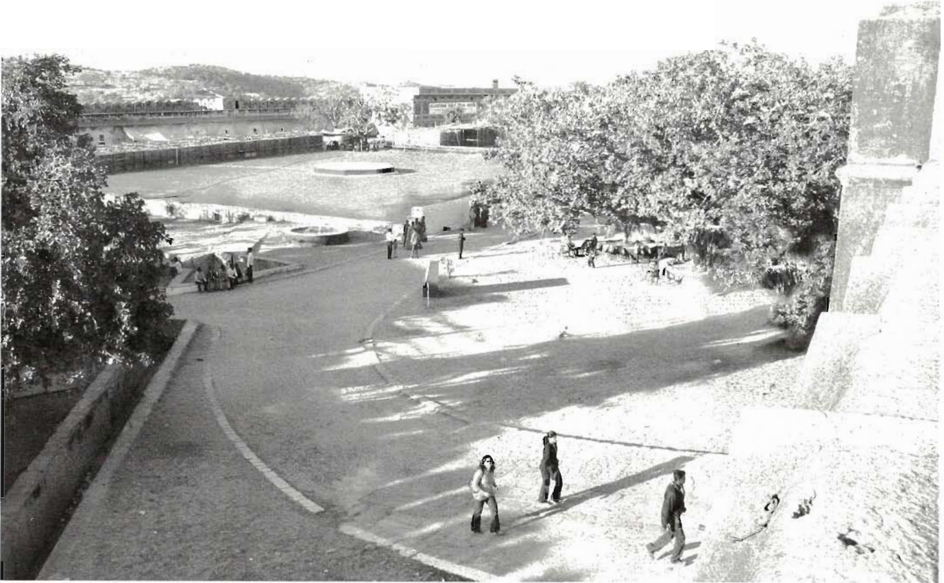
Fig. 9.10C. Diversion swale (channel entering from lower left corner) directs water to enter a covered cistern in Jaipur Fort, India. Uncovered cells or square tanks (see people sitting at edge of the tank) capture the silt in the runoff, and the slope of the diversion swale itself is greatly reduced so silts settle out and relatively silt-free water enters the massive cistern (beneath square plaza-like cover with raised octagon in its center).
