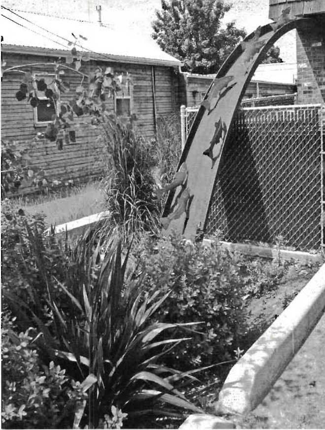
5.29. Celebrate the rain! Steelhead trout swim up a steel downspout directing roof runoff to a rain garden below. Portland, Oregon. For color photo see inside front cover
