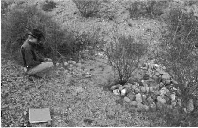
Fig. 10.37. Chet Phillips inspects a check dam holding a level terrace of soil high in the Teran watershed.
