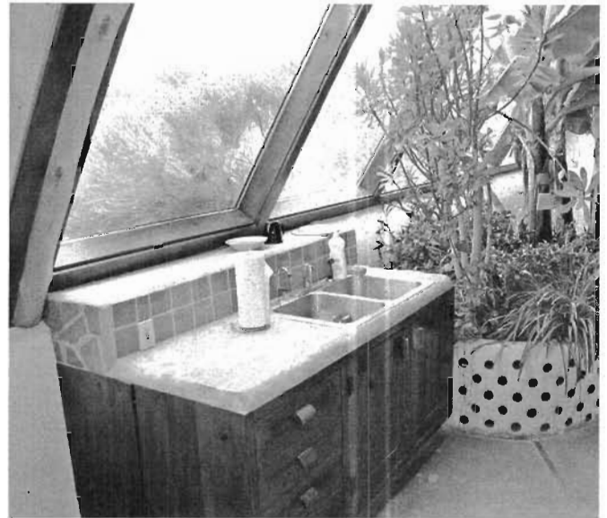
Fig 12.8. Greenhouse greywater harvesting in cold climates. Sink water drains to the adjoining planting bed to irrigate bananas and more at the Earthship Visitors Center in Taos, New Mexico.
