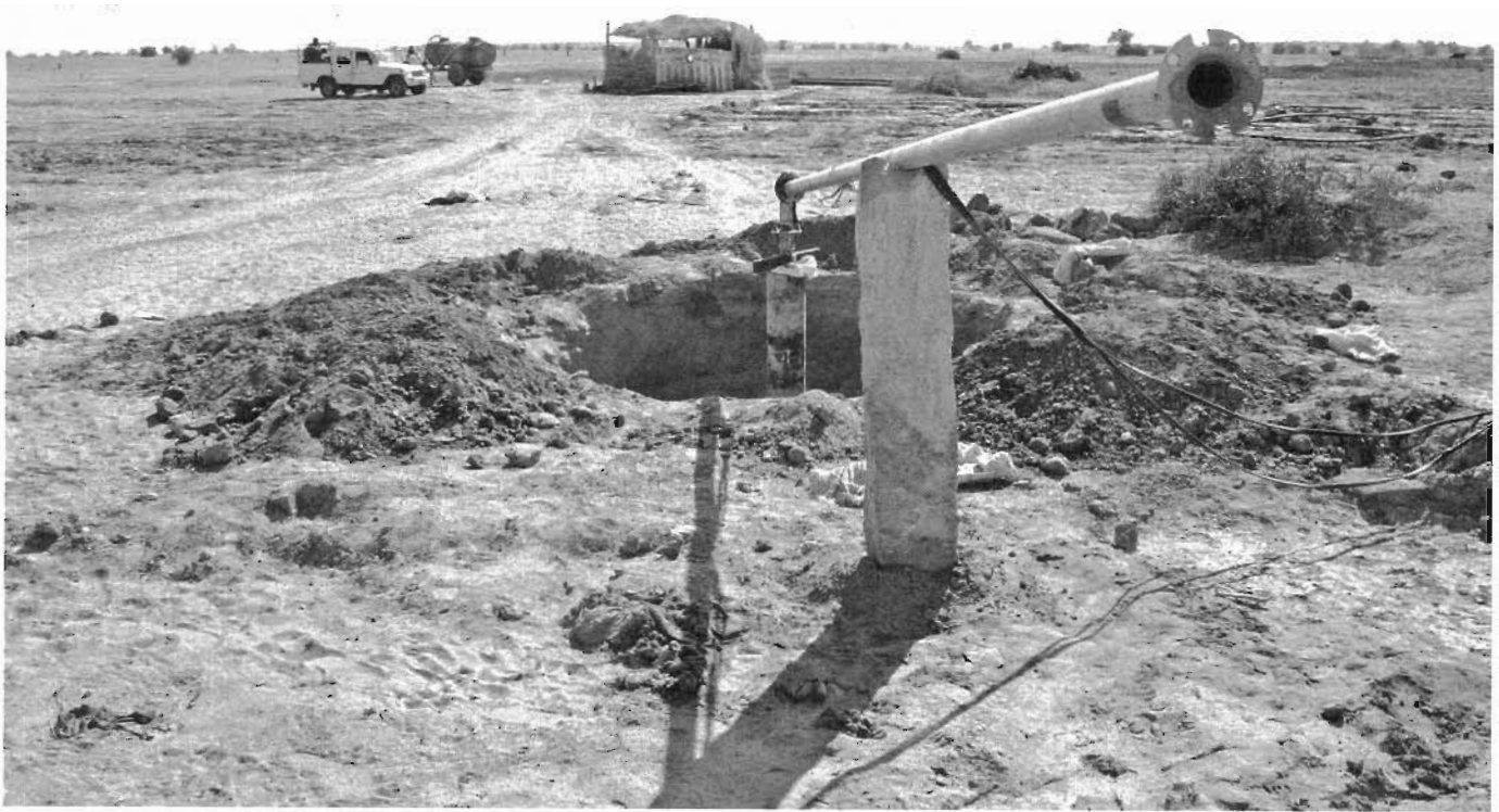
Fig. I.9. This well and the field in background were abandoned after groundwater was depleted and irrigation with pumped groundwater raised salt levels in the soil to the point that plants would no longer grow. Jaisalmer District, Rajasthan, India.
