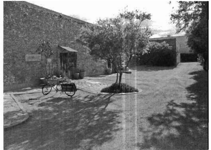
Fig. 8.15A. Porous-aggregate parking lot and salvaged-concrete walkway, Tucson, Arizona. Note: The system could be improved if walkways directed their runoff to vegetated basins rather than the parking lot.
