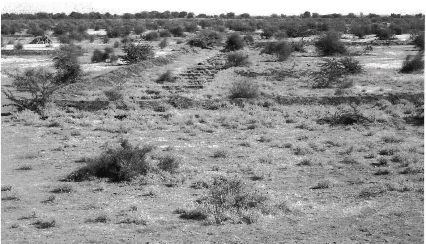
Fig. I.18. Sahalsagar choukas. Slope is from right to left. Chouka in the background overflows to the chouka in the foreground, which overflows to another series of choukas downslope to the left.
