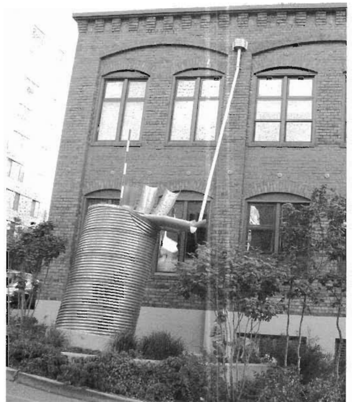
Fig. 3.22. View of the Beckoning Cistern from across the street. A faucet enables neighborhood gardeners to utilize the cistern water to irrigate the adjoining plantings.
