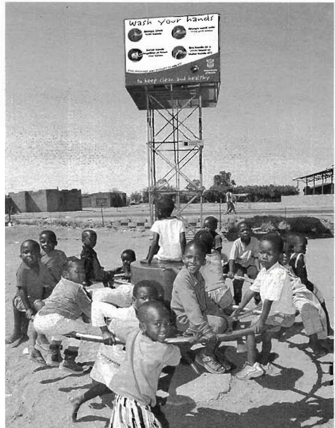
Figure A6.1. Children playing on a PlayPumps merry-go-round provide the power to pump groundwater into the raised water tank for gravity-fed distribution. The advertisement signs around the tank help pay for the system. Courtesy of PlayPumps International. www.playpumps.org .
