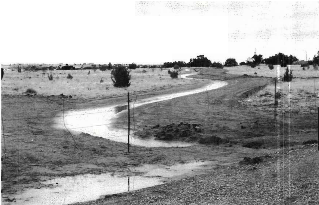
Fig. 9.23. Diversion swale harvesting runoff
