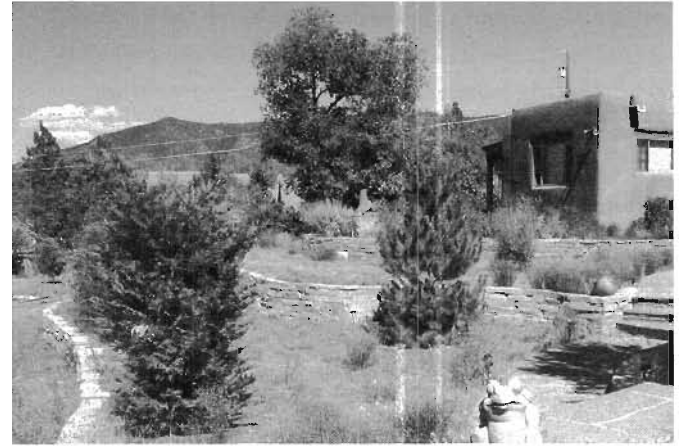
Fig. 3.8. Terraces with sandstone retaining walls built by Raincatcher and San Isidro Permaculture harvest direct rainfall in Santa Fe, New Mexico. Although unseen, there is beneficial water-harvesting redundancy here. Roof runoff from canales (roof drains) is stored in an underground cistern and distributed via an automatic drip system to irrigate vegetation in dry times. A greywater system (shower, sinks, and clothes washer) adds additional irrigation water via French drains with perforated pipe.
