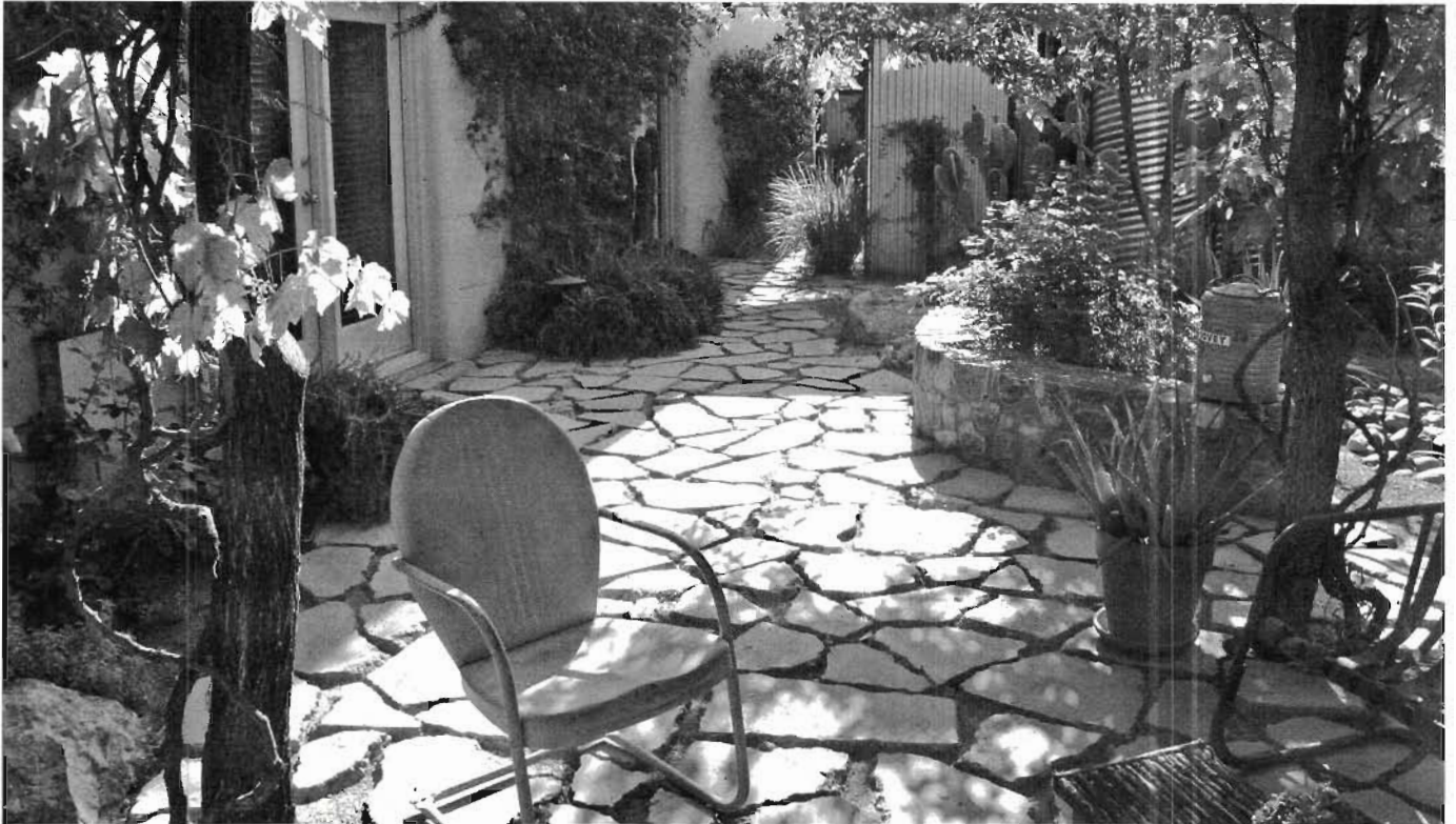
Fig. 8.19. Salvaged chunks of concrete sidewalks are decoratively laid as a porous patio in the award-winning landscape of the Amado residence, Tucson, Arizona. Designed by Blue Agave Landscape Design
