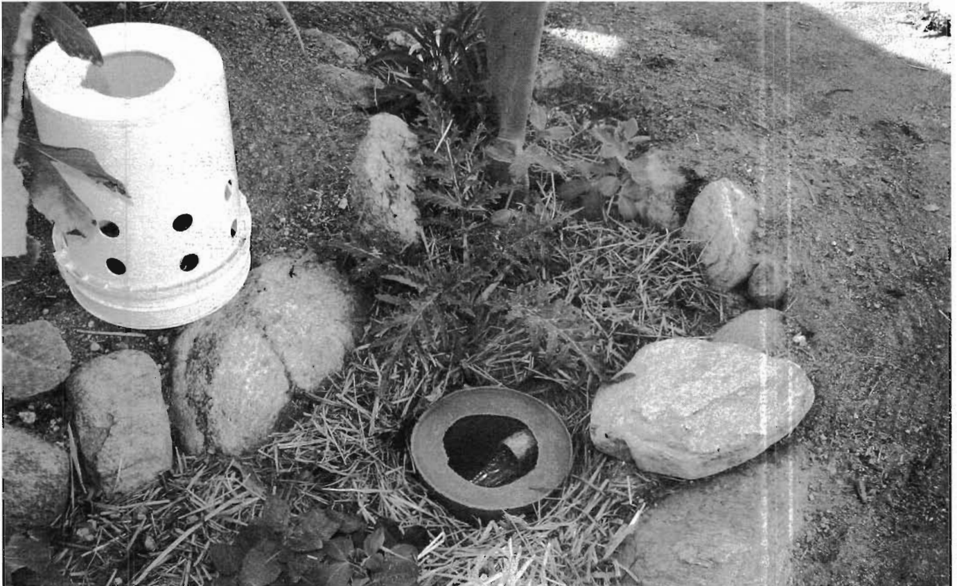
Fig. 12.11. A greywater drain discharging into a mulched basin via a subsurface outlet shield made from an upside down 5-gallon (19-liter) plastic bucket with holes drilled into its sides. An unused bucket outlet shield sits beside the basin to illustrate what the bucket within the basin looks like. Note: The hole cut in the bottom of the bucket (which is the top of the shield) is smaller in diameter than the bucket bottom, leaving a rim of plastic that keeps the bucket firm and strong. WARNING: The outlet shield must be placed within a much larger mulched basin sized to handle the peak surge of greywater entering it. That way greywater flowing out of the shield is fully contained and quickly infiltrates, as seen here. A bucket shield without an associated mulched basin is too small to adequately infiltrate greywater surge, and will lead to smelly anaerobic soil conditions. The flat rock seen here sitting beside the drain outlet is placed over the chamber to prevent the plastic from degrading in the sun, to improve appearances, and to keep the greywater below the surface of the rock and mulch. The mulched basin also harvests rainwater from the surrounding area. The rock that lines the basin banks stabilizes the basin's edge.
