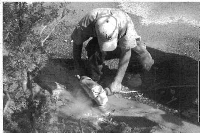
Fig. 8.36. Smoothing out the cuts and edges with an industrial hand-held grinder
