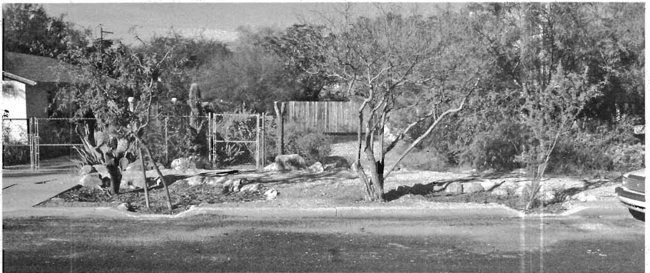
Fig. 8.37. The finished curb cuts, basins, and trees permitted with the drawings from figs. 8.34A, B. Note that the less drought-tolerant tree between the basins will be removed once the two food-producing native trees in basins grow to a larger size.
