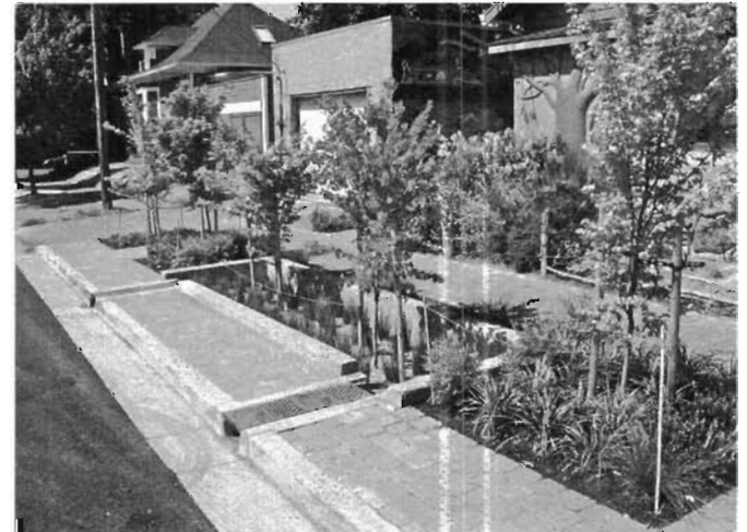
Fig. 8.27. Curb cuts along a residential street beside the People's Co-op, Portland, Oregon. Sidewalk strip beside curb allows for easy access of people entering and exiting cars parked along curb, while steel scupper directs runoff water to vegetated infiltration basin. Raised curb alerts pedestrians to edge of basin.
