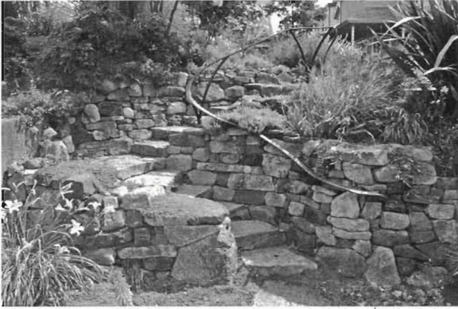
Fig. 3.2. Terraces stabilized with dry-laid stone walls and accessed via a whimsical stairway. Stonework by Goettling McGee, Inc., Seattle, Washington
