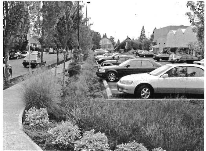
Fig. 8.29. Water-harvesting parking lot, New Seasons Market, Portland, Oregon. Parking area drains to adjoining sunken, mulched planting areas. Wheel stops keep cars out, but let water pass by. Trees are planted on slope so their roots can access the harvested water, while their root crown is well drained. As trees grow, they will canopy over the asphalt.
