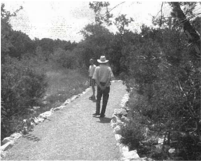
Fig. 2.7. Raised path with rock-stabilized edges, Lady Bird Johnson Wildflower Center, Austin, Texas
