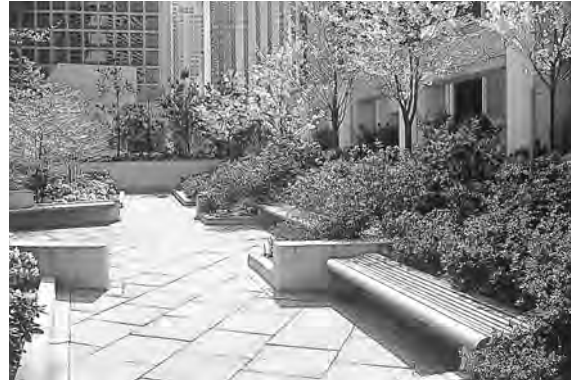
Plate 188 If raised planters are to include standard trees, a generous width is desirable because this allows good capture of natural precipitation (Union Square, Seattle, USA).
