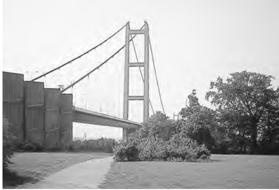
Plate 117 The largest structures in the landscape, such as the Humber Bridge, near Hull, UK, require plantations and tree clumps of generous size to maintain good generic scale relationships.
