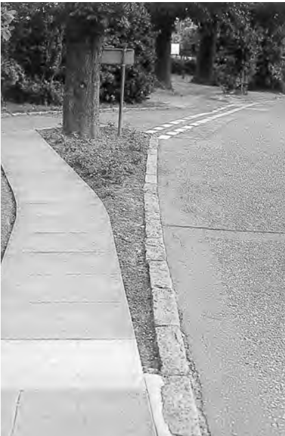
Plate 176 Narrow planting beds do not provide adequate soil conditions and are vulnerable to trampling.
