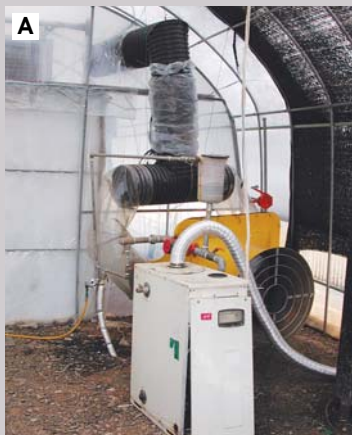
Figure 13. Equipments for environmental management A: Boiler B: Duct
