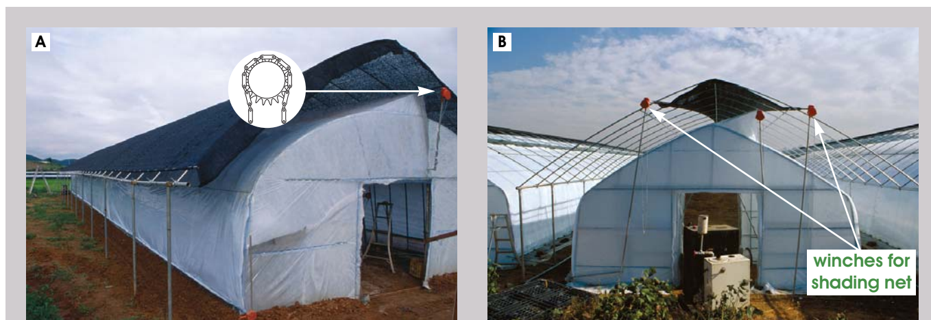
Figure 6. A: Outer structure and shading net B: Shading net rolled up
