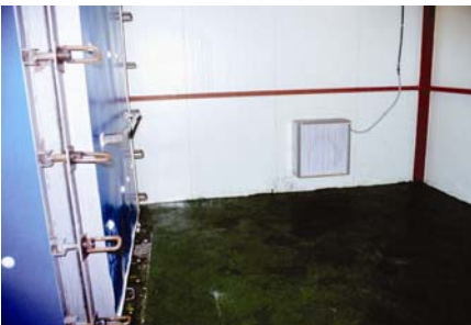
Figure 10. Autoclave door to the pre-cooling room
