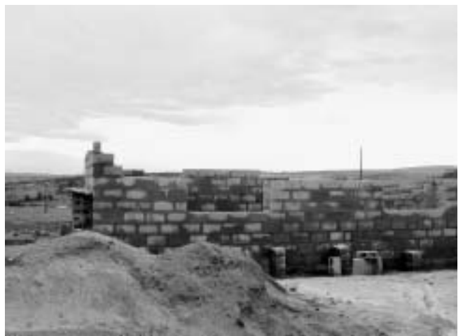
Figure 22. Mushroom center for storage, packing, processing (under construction)
