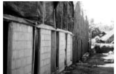
Figure 9. Steam pipes on the brick wall
